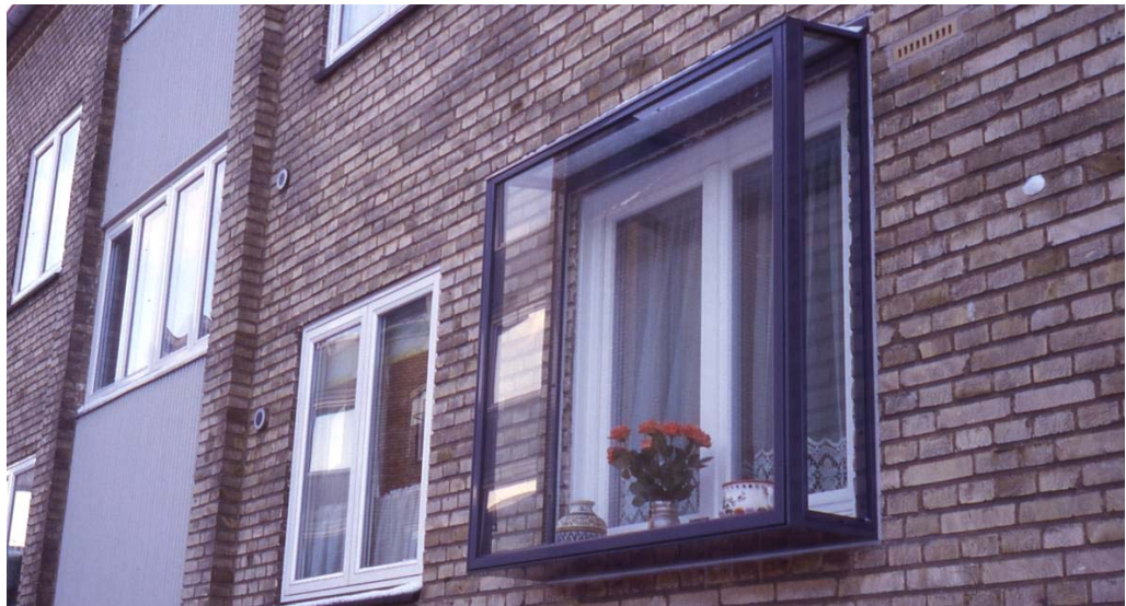
Figure 1.1. Façade insulation by applying a “glass box” in front of an existing window of bedroom or living room. Example from an apartment building in Århus, Denmark [10].
