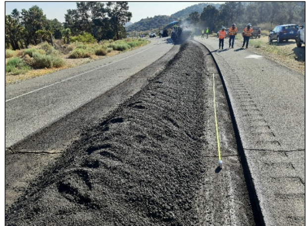
Figure 4.6: SBD-2: Spacing of transverse cracking.
