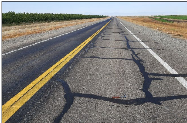
Figure 2.1: GLE-162: Alligator B cracking.
