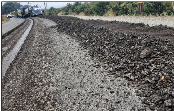
Figure 3.17: SB-135: Oversize RAP from incorrect pre-milling speed.
