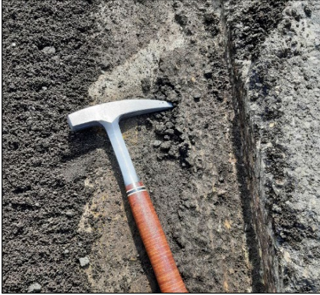
Figure 3.13: SB-135: Recycling depth at the interface between two lifts.
