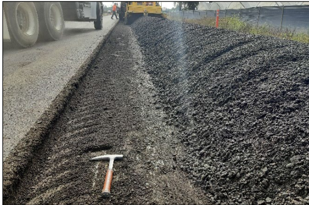
Figure 3.15: SB-135: Layer of fine material in the cut next to the windrow.
