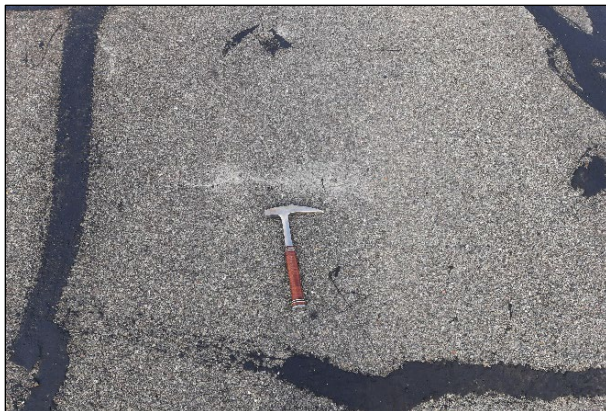
Figure 2.3: GLE-162: Pumping of fines through unsealed cracks.
