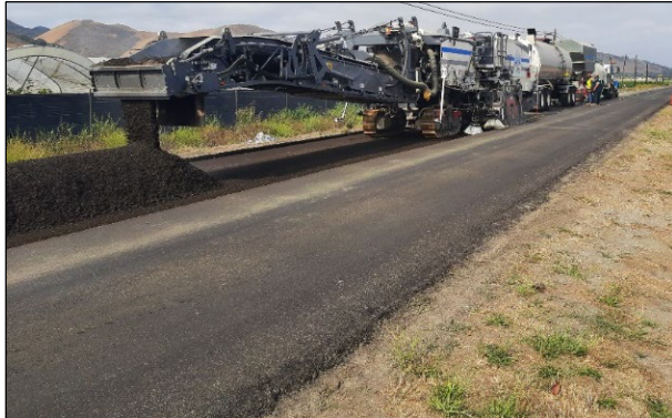
Figure 3.8: SB-135: Single-unit recycling train. (Water tanker and cement spreader, asphalt tanker, recycling unit).
