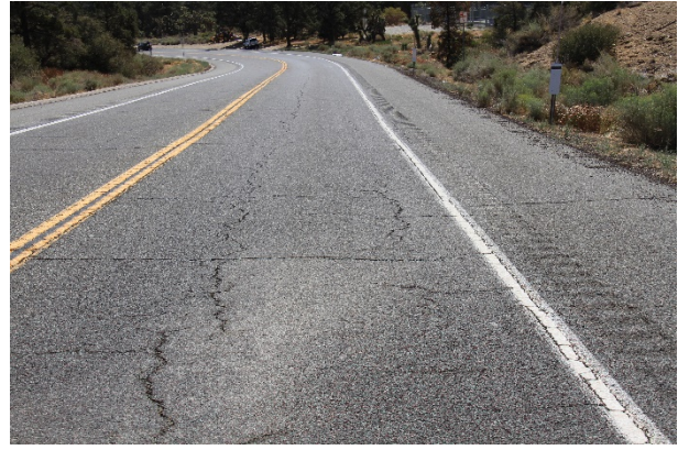
Figure 4.2: SBD-2: Block cracking.
