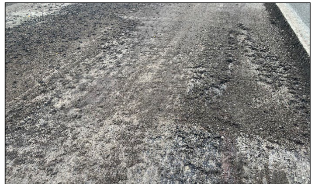
Figure 4.8: SBD-2: Remains of asphalt rubber chip seal SAMI at bottom of milling cut.
