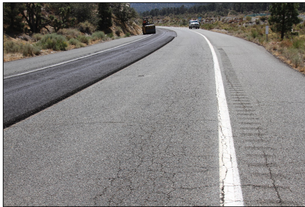
Figure 4.3: SBD-2: Alligator B cracking in the wheelpaths.
