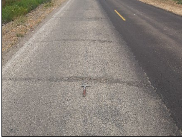
Figure 3.3: SB-135: Transverse cracking.
