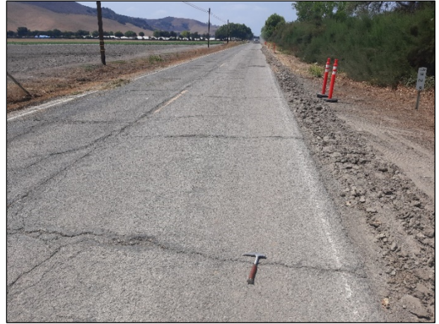
Figure 3.4: SB-135: Spalling on cracks.
