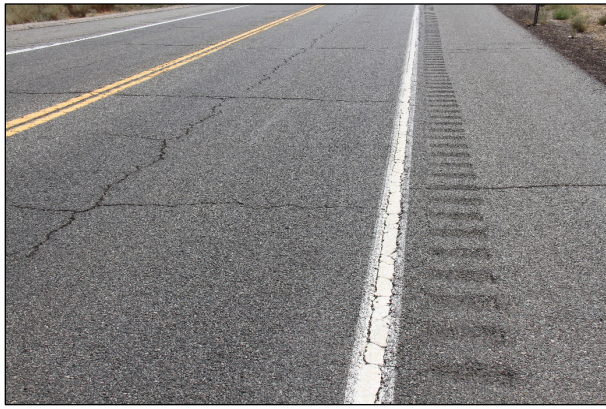
Figure 4.1: SBD-2: Transverse and longitudinal cracking.
