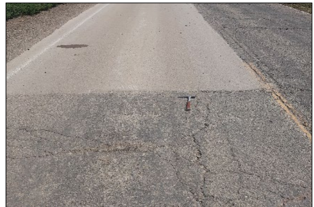
Figure 3.2: SB-135: Lane-width patches.
