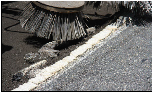
Figure 4.7: SBD-2: Material from centerline and shoulder cracks collapsing into cut.
