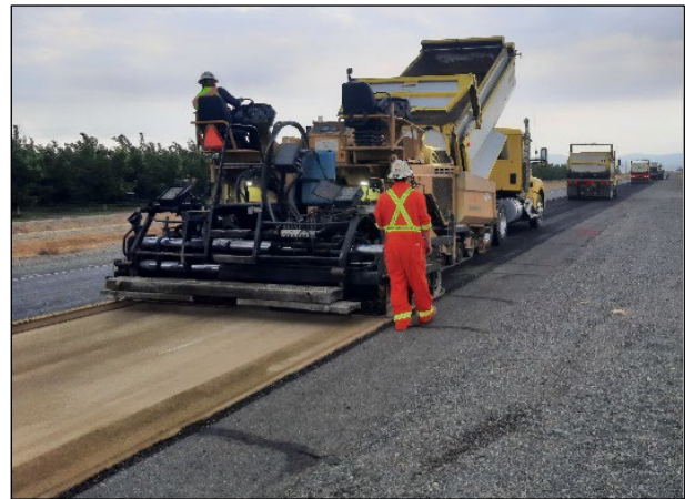
Figure 2.19: GLE-162: Paving supplemental rock dust material.
