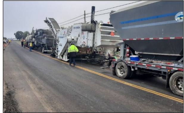
Figure 3.9: SB-135: Multi-unit recycling train. (Water tanker and cement spreader, milling machine, crushing and processing unit, asphalt tanker).
