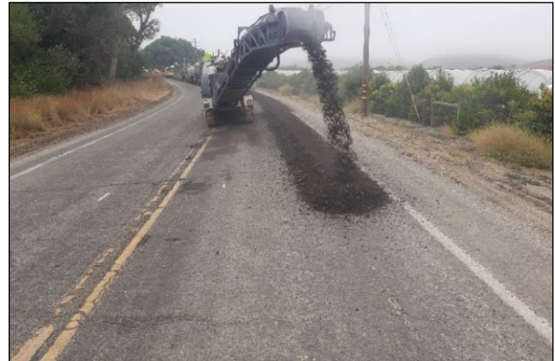
Figure 3.16: SB-135: Milling machine in front of recycling train.
