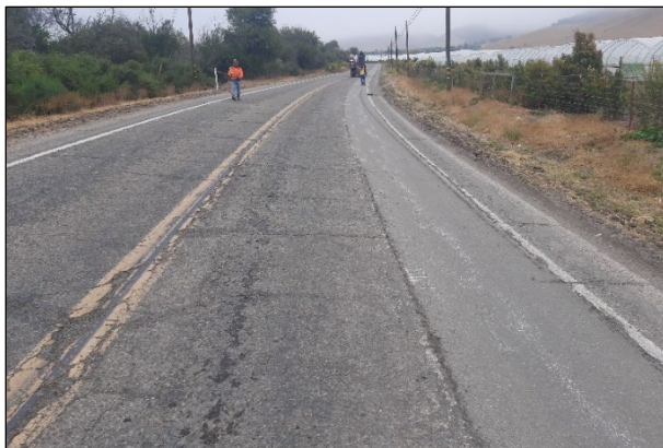
Figure 3.1: SB-135: Wheelpath patches.
