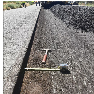
Figure 4.11: SBD-2: Aggregate base next to old asphalt concrete in cut.
