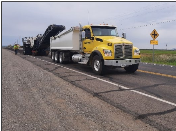
Figure 2.18: GLE-162: Pre-milling in front of the recycling train.
