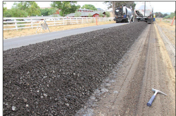
Figure 3.12: SB-135: Native soil in outer 1 ft. (0.3 m) of recycle cut.
