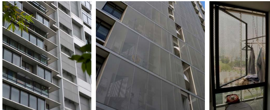
Figure 9. Multiple exterior shading types in Moulmein Rise Residential Building, Singapore by WOHA Architects. left: south façade. middle: north façade. right: view out the north façade. Images from < archnet.org > and < www.akdn.org >
