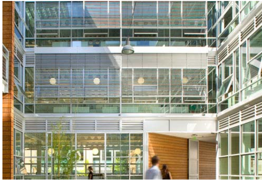
Figure 41. (Left) Terry Thomas Building has awning windows behind exterior venetian blinds. Image from <www.weberthompson.com>. Figure 42. (Right) Window opening types tested. (Chandra 1986)
