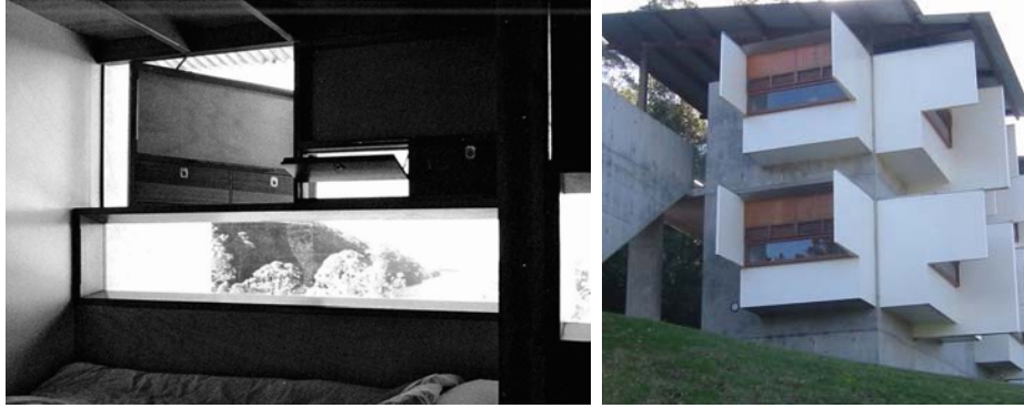
Figure 20. Compound windows with multiple operation types within the same opening. Left and middle, Boyd Educational Center, Glenn Murcutt, 2005. -34.8°S latitude. Illaroo, NSW, Australia. Image from Dahl, 2010.
