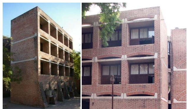
Figure 4. The IIM Dormitories in Ahmedabad, India (Louis Kahn) were designed to be protected from the sun and permeable to the wind. Images from < www.flickr.com/photos/jmordhorst/ > and < www.flickr.com/photos/12474755@N07 >
