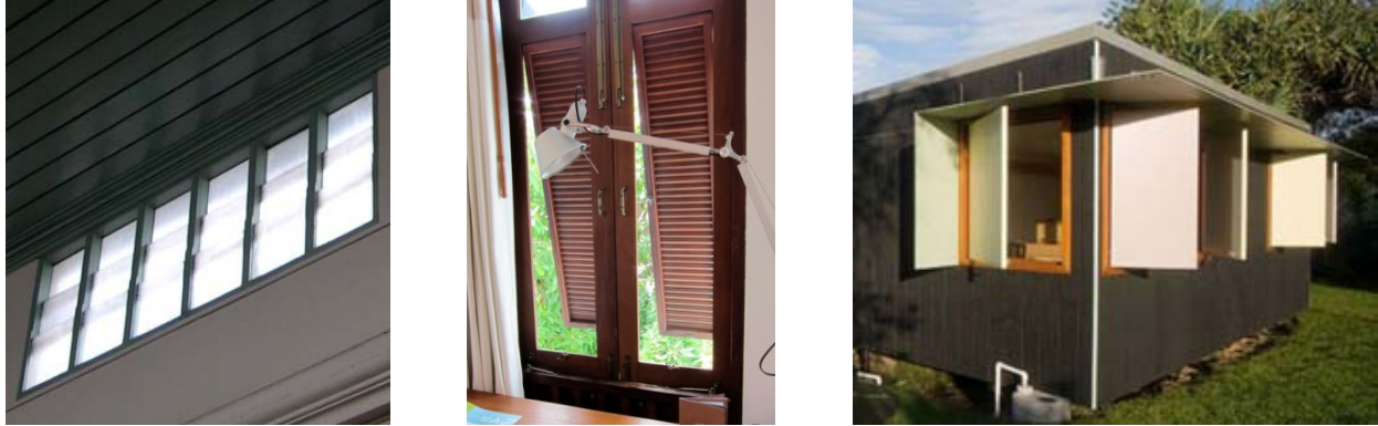
Figure 3. Left: A rare use of staggered fixed pane glazed windows allow for the passage light and air while blocking rain. Wat Phra Kaeo Museum. (photo by author). Middle: dual action windows with panel sashes that can open like a double casement or like awning windows or “Bahama shutters” at Let’s Sea Hua Hin Resort, Thailand. Window sashes, when present in the tropical vernacular, tend to be solid or slatted shutters. (photo by Sittha Sukkasi). Right: Overhangs and solid panel casement windows in Happy Haus in Queensland, Australia 6
