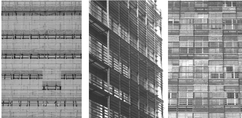
Figure 21. Screen shading systems are prevalent in contemporary architecture. From left to right: perforated panels, thin louvers and wood slats.
