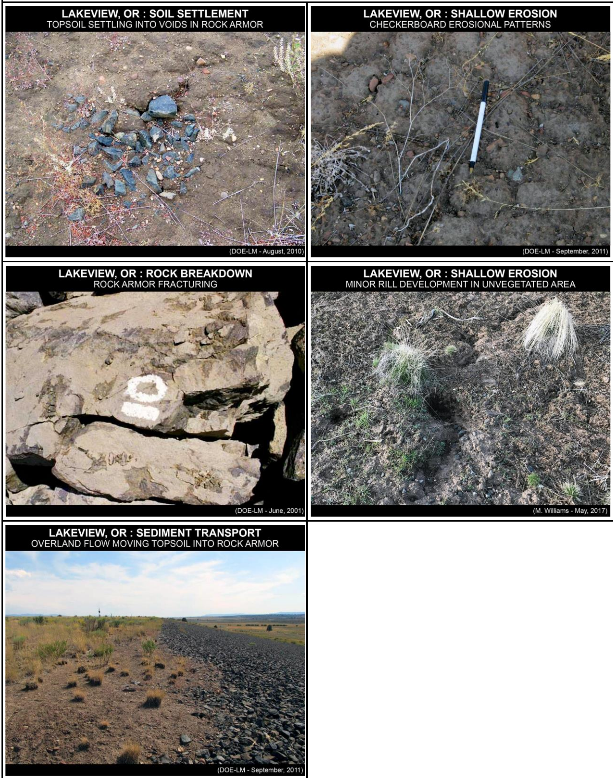
Figure A.9. Lakeview, OR : Surface Features Characteristic of Geophysical Processes
