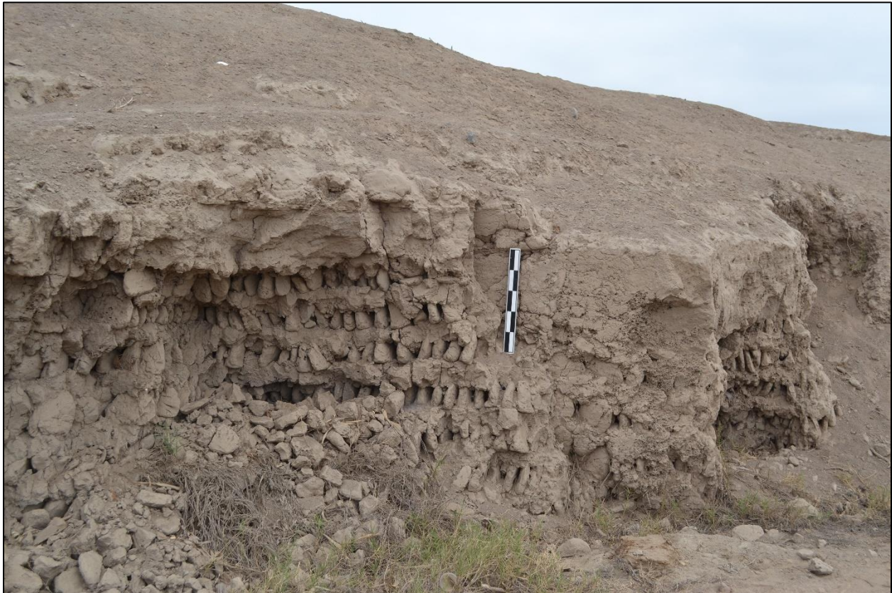
Figure 11: Exposed substructure at PV57-25 (Huaca Soto West) showing conical adobe units laid into coursings and sealed with mud-slurry caps.
