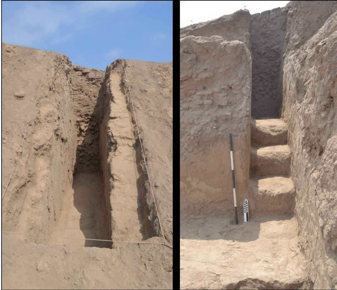
Figure 54: Narrow access corridor in the northeastern corner of Sector A. The image on the left is from the exterior atrium looking towards into the court. The image on the right is from the second internal tier of the court looking outward towards the atrium.
