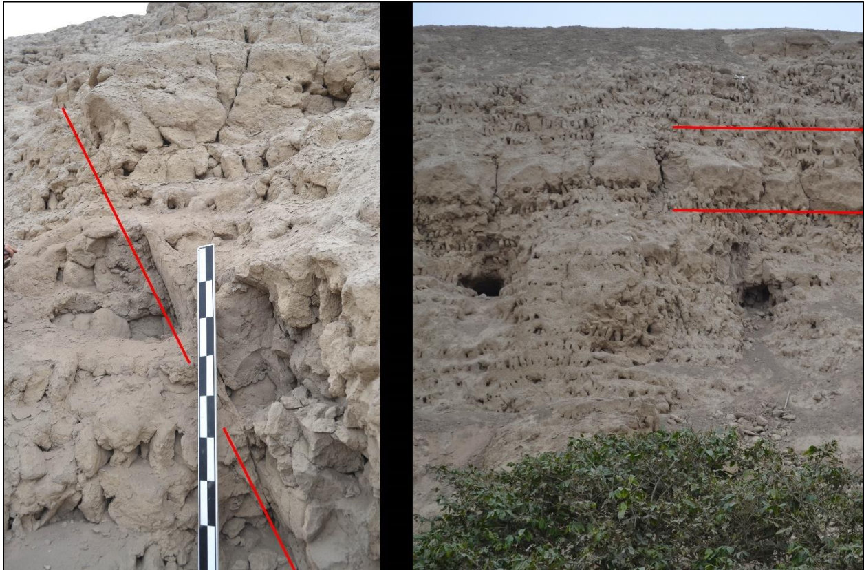
Figure 40: Structural anomalies in Huaca Soto's exposed western end. At left, marked by a red line, is a long finished 'seam' embedded in the masonry sections of Huaca Soto's western face. At right, marked by two horizontal lines, is thickened mud cap with no internal adobes.
