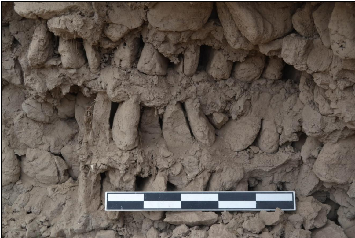
Figure 39: Paraboloid adobes and mud-slurry caps in situ within the exposed western face of Huaca Soto.
