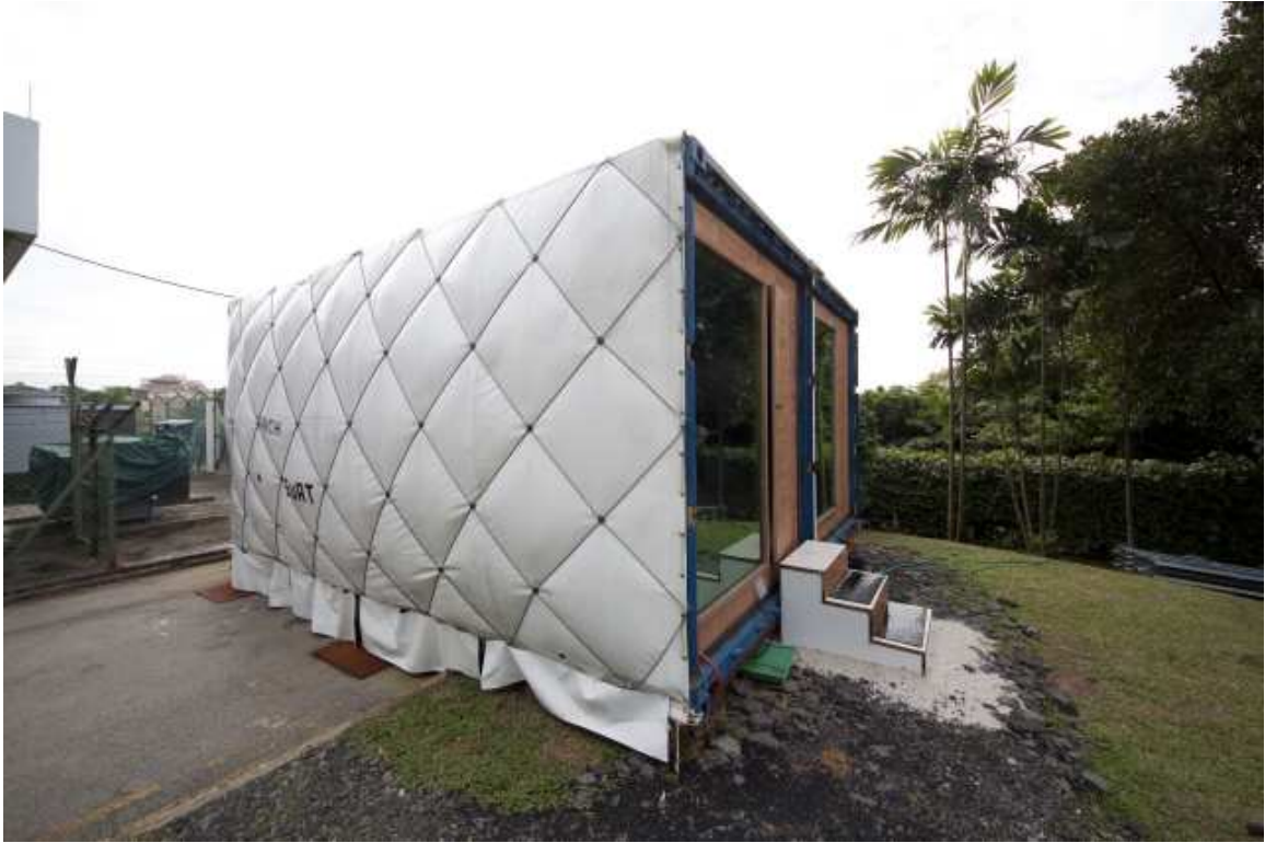
Figure 5.6: BubbleZERO test-bed owned by Future Cities Lab of ETH Zurich, and located on the campus of National University of Singapore.
