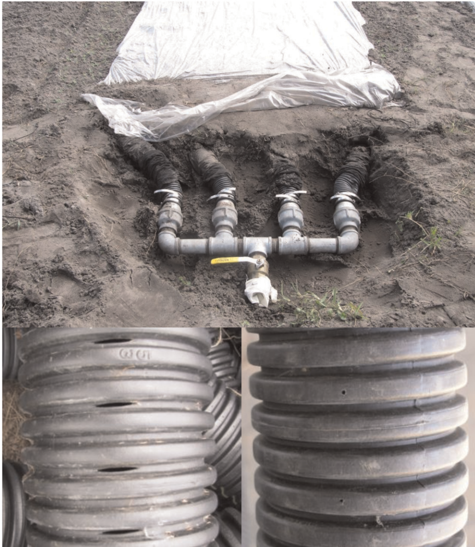
FIG. 1. Perforated medium density polyethylene plastic pipe (7.6 cm diameter) used with saturated steam. This method is well suited for combined use with solarization, and is relatively efficient with regard to fuel consumption. Four pipes were installed in each planting bed, with at least one pipe per foot of bed width. Pipes were laid in trenches at 35-cm depth with the objective of heating the top 20 cm of soil. Lower right: standard 7.6 cm perforated plastic drain tile (steam 1), lower left: custom-drilled plastic drain tile with 1.6-mm holes spaced every 3.8 cm (steam 2).
