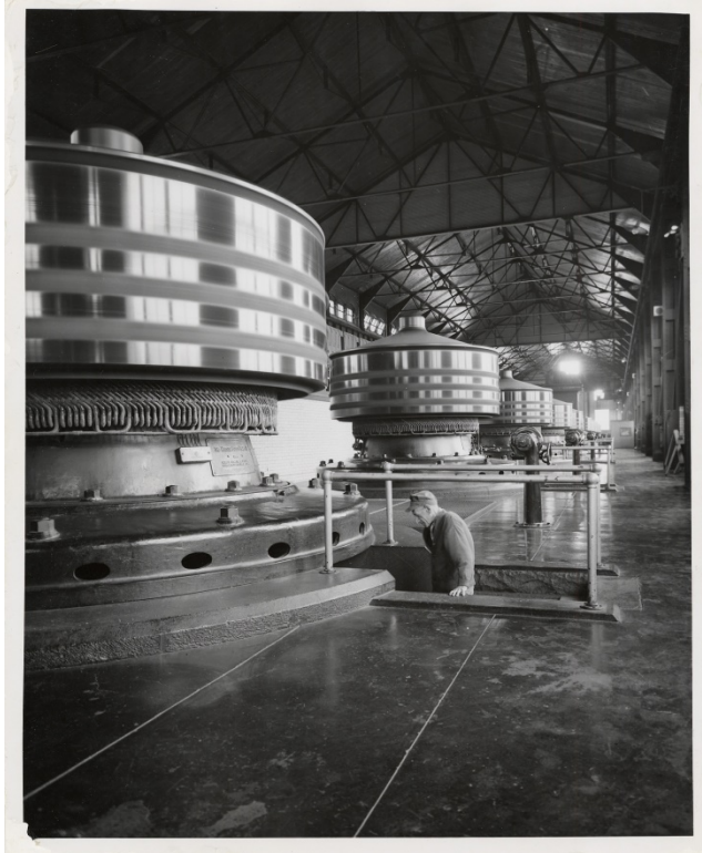
Figure 3 Westinghouse/Tesla generators at Niagara Falls (See Image Note 3)
