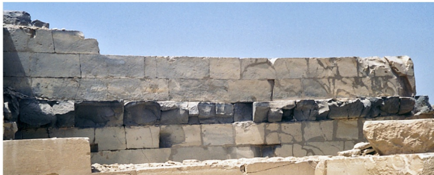
c. bituminous limestone (var. 1) used in a wall in the pyramid temple of Pepy I, Dynasty 6, at Saqqara, Egypt.
