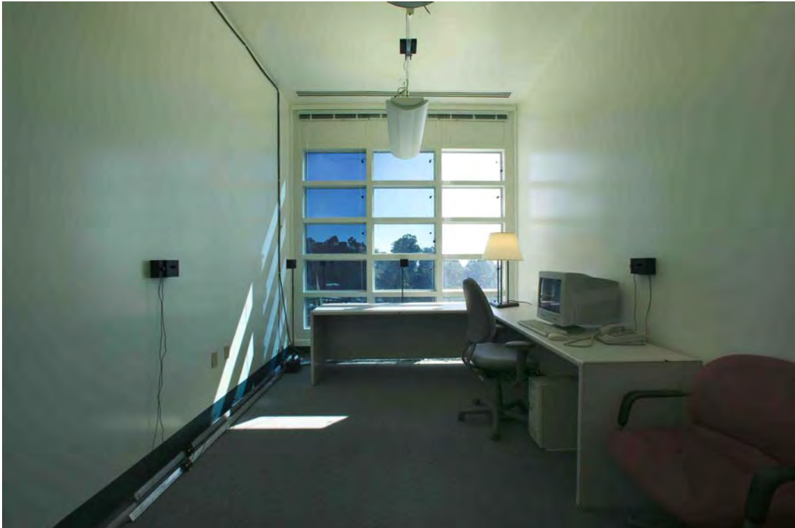
Figure 11. Interior view of EC window wall shortly after EC windows were first installed, September 10, 2003.
