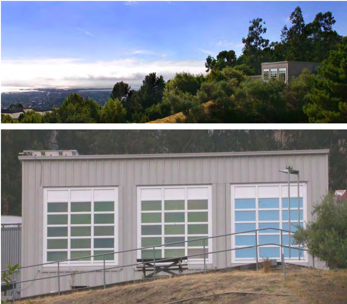
Figure 2. LBNL Window Testbed Facility (upper photo). South elevation of EC facades (middle and left) and spectrally selective low-e façade (right) on August 20, 2004 (lower photo).
