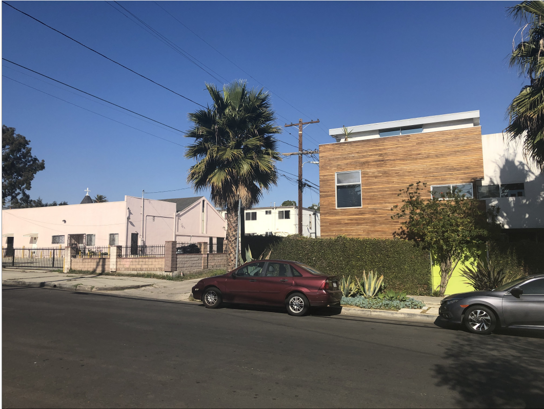
Figure 2.3: Friendship Baptist Church (left) and New Construction, Venice, 2020
