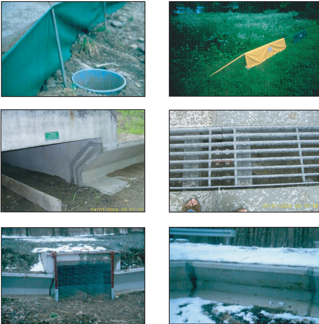
Figure 8. Mitigation measures for amphibians in Poland (top left: detail of a temporary mitigation measure at Via Baltica S8. Note that the bucket was dug in farther away from the fence and amphibians can pass it. Also, the pole should have been fixed on the other side of the fence not to disturb amphibian movement. top right: Frog King type of amphibian fence; middle left: tunnel entrance with guiding structure; middle right: concrete amphibian fence element from above built in where a small side road joins the main road; bottom left: entrance of an amphibian tunnel at Jeleniow; bottom right: concrete fence element at Jeleniow)
