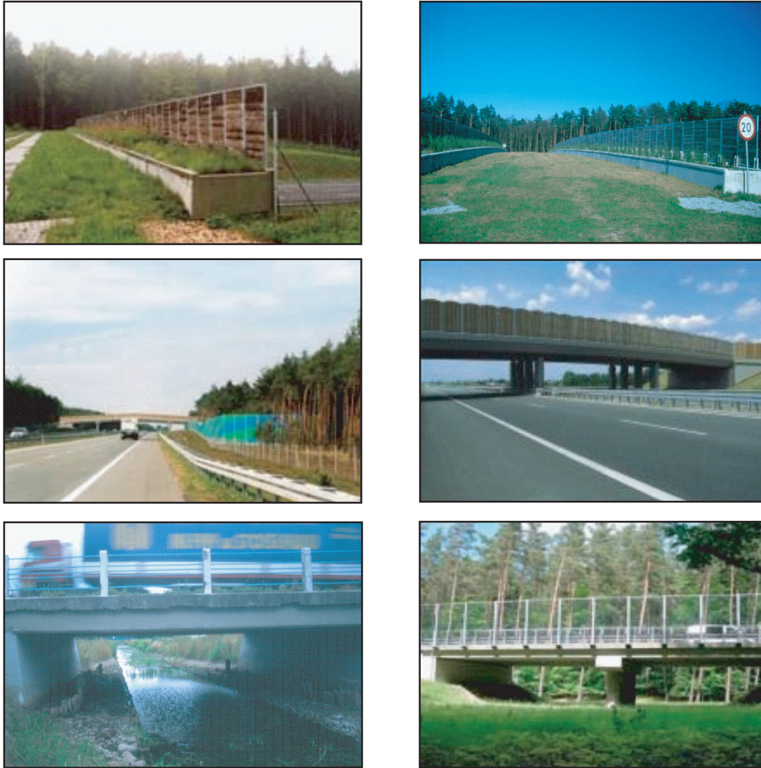
Figure 7. Game bridges and wildlife passages in Poland (top left: Multifunction (animals, agriculture) fauna bridge on A4; top right: Multifunction (animals forestry) fauna bridge on A4; middle left: Guiding lines of fauna bridge on A2; middle right: Fauna ridge on A2; bottom left: underpass for Lutra lutra (Kampinos National Park); bottom right: Underpass for big and medium mammals on expressway no. 3).
