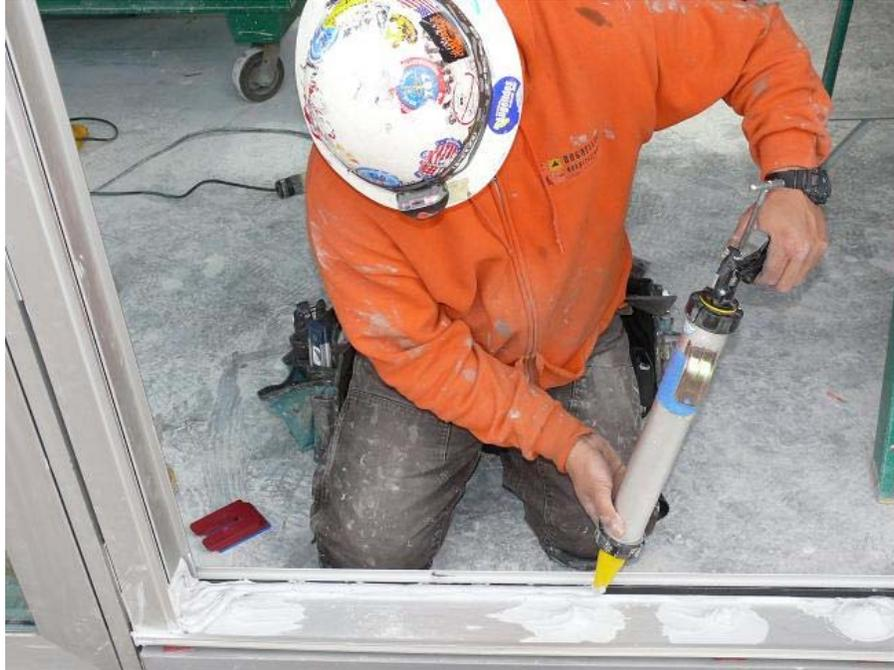
Figure 5.15 Worker applying silicon paste to bottom sill
