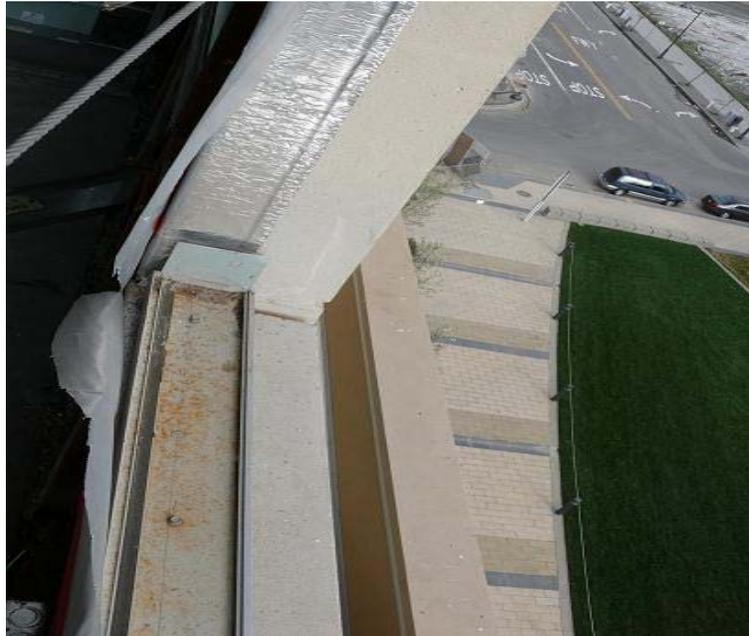
Figure 5.4 Bottom sill installed on the Glass Fiber Reinforced Concrete (GFRC)
