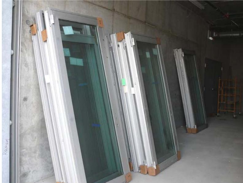
Figure 5.11 Windows unpacked and sorted according to their corresponding floors
