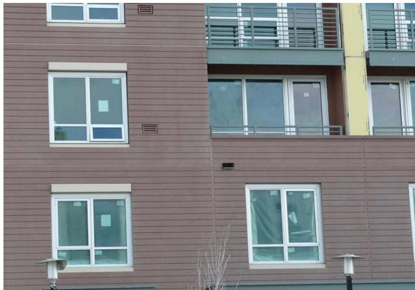
Figure 5.3 Dual glazing projected windows in Project X
