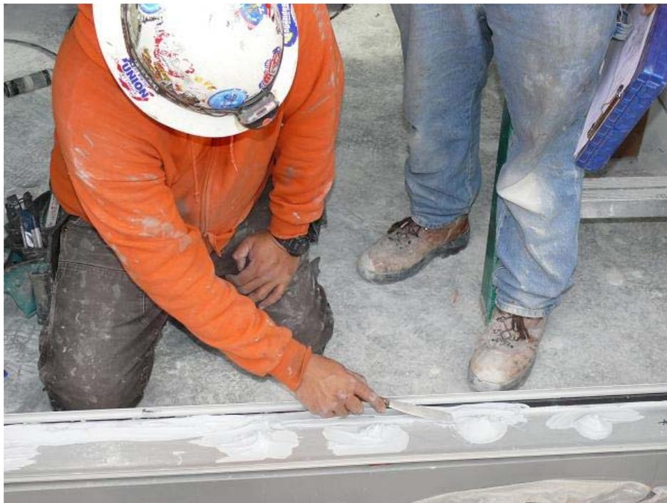
Figure 5.16 Worker smoothing the silicon paste to remove possible air bubbles
