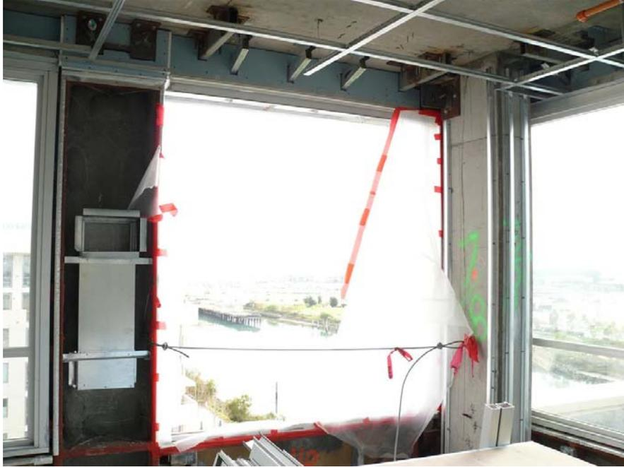
Figure 5.13 Window opening cleared for installation
