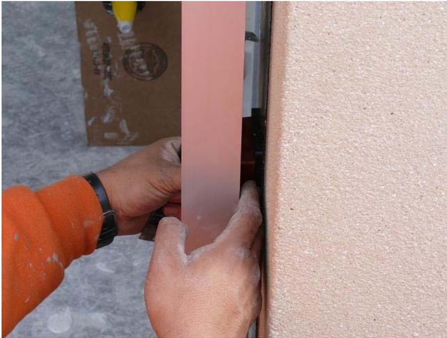
Figure 5.14 Plastic spacers placed behind the aluminum frame to adjust and space the gap between the uneven concrete and the aluminum frame
