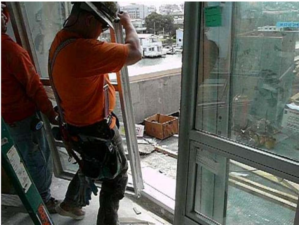
Figure 5.18 Two workers lifting a window pane and placing it on the frame
