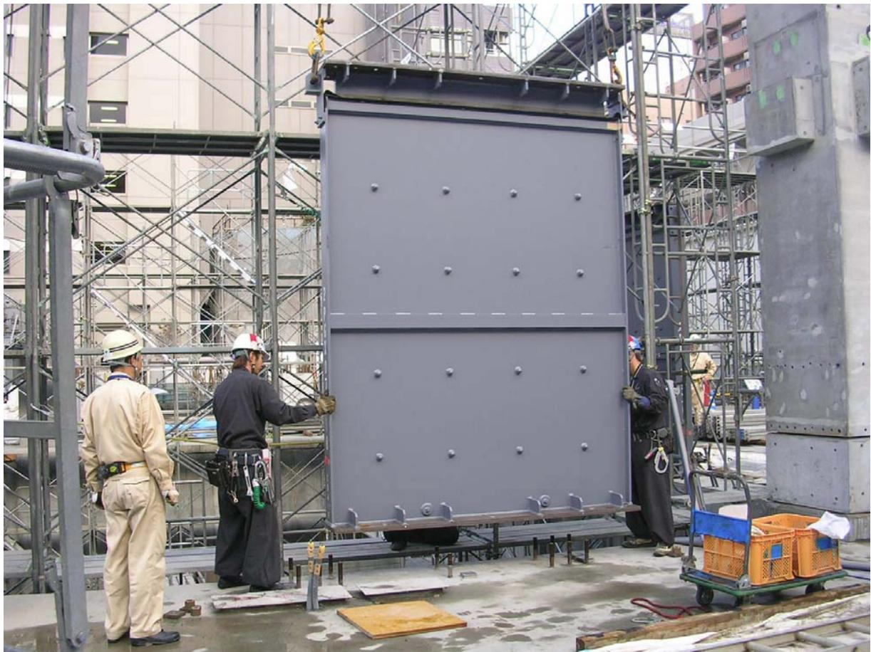
Figure 6.3 VDW installation on concrete structure using sequential installation method in Japan (courtesy of DIS)
