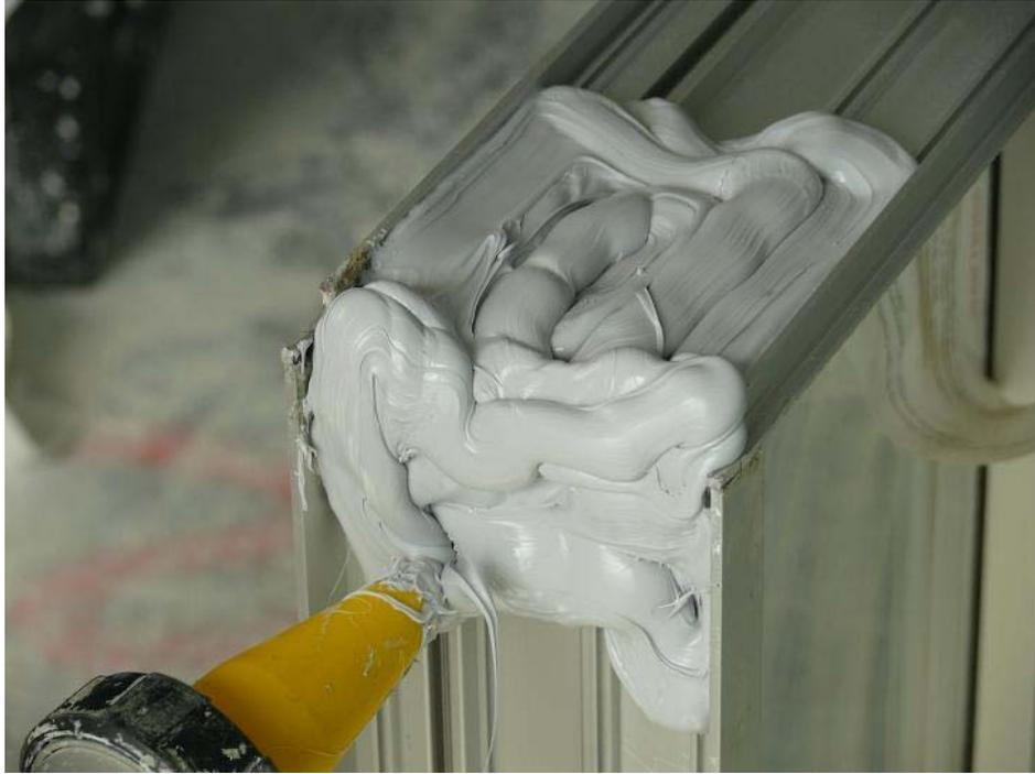
Figure 5.17 Worker applying silicon to window frame
