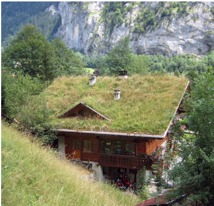
Figure 6. This vegetative (green) roof covering provides Class A protection in terms of fire penetration into the attic or living space, but ember ignition and subsequent flame spread and contact with the dormer and window shown in this photograph could result in the glass breaking and fire entering the building. Photo: Bernard Harrison.
