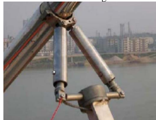
(c) MR dampers installed on Dongting Lake Bridge
