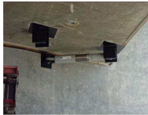
(b) Viscous fluid damper on 91/5 Overcrossing
