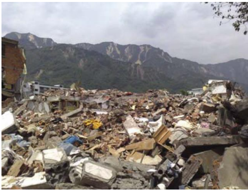
(a) Complete destruction of four buildings
