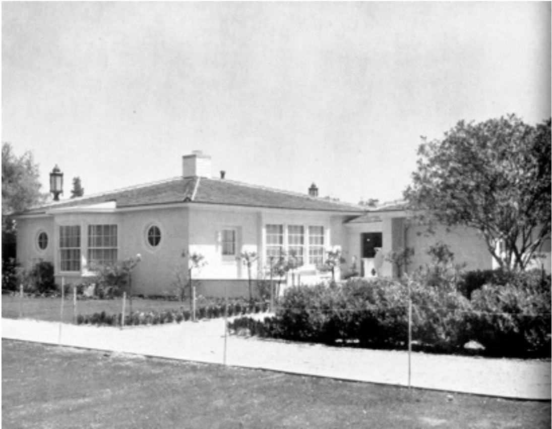
Figure 37. Winchton L. Risley, California Cottage, Los Angeles, 1936.
