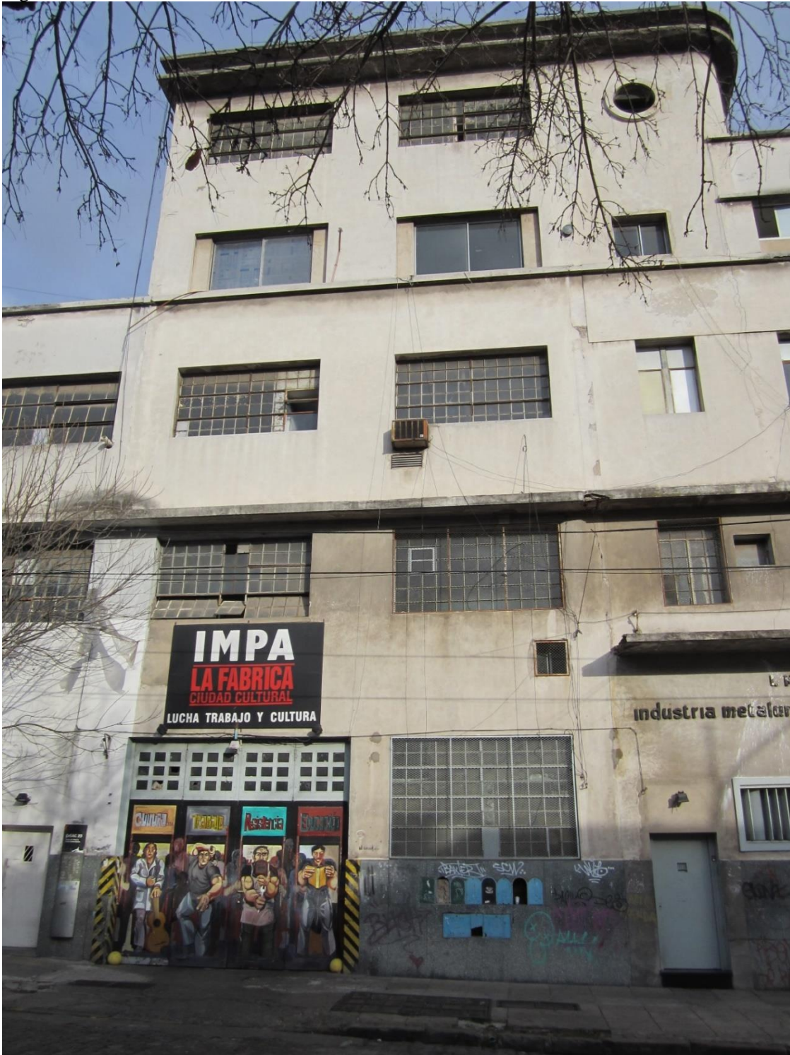
The sign reads: "IMPA: The Factory: Cultural City: Struggle Work and Culture." The four panels read: "Culture, Work, Resistance, Education."
