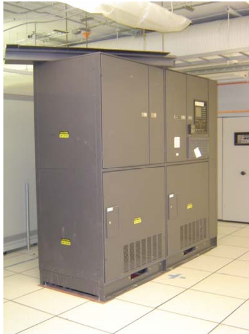
Figure 9. Typical PDU
