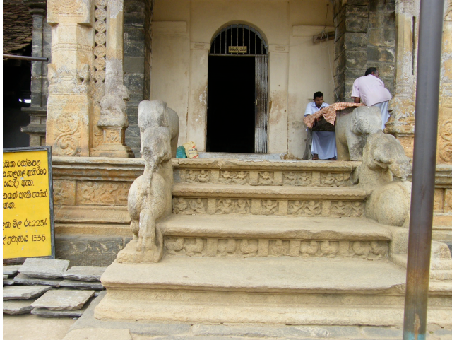
Fig. 2.4. Carvings on Entrance Staircase, Gadalâdeniya
