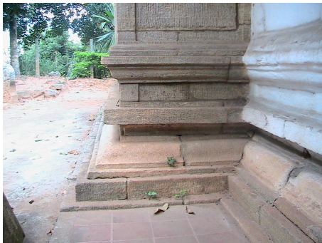
Fig. 2.37. Basement moldings, Âdahana Maluwa
