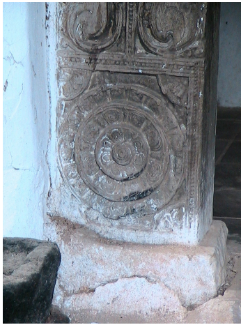
Fig. 4.54. Detail of wooden doorway, Simhâsana, Soragune Devâle
