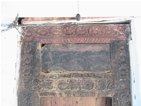
Fig. 4.42. Lotus motif on lintel, Shrine to the deity Kataragama, Soragune Devâle
