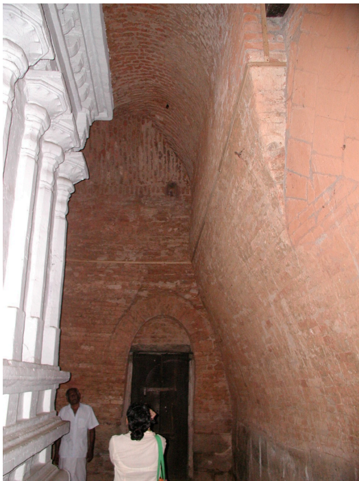
Fig. 2.46. Basement moldings and exterior wall of inner sanctum, Lankâtilaka
