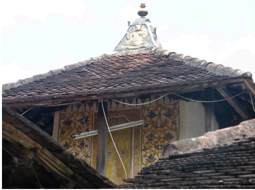
Fig. 4.9. The second storey of the inner sanctum, Embekke Devâle
