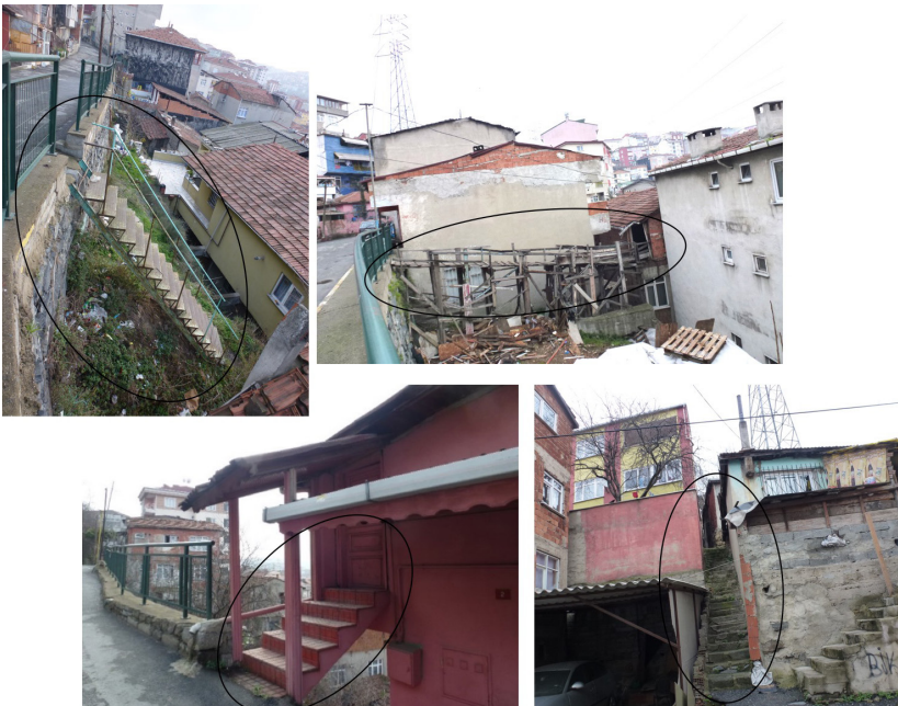
Figure 8 Connections Between Houses and Roads (Photos by authors)
