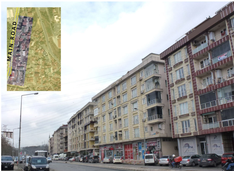
Figure 6 New Buildings after Transformation in the Area (Photo by the authors)
