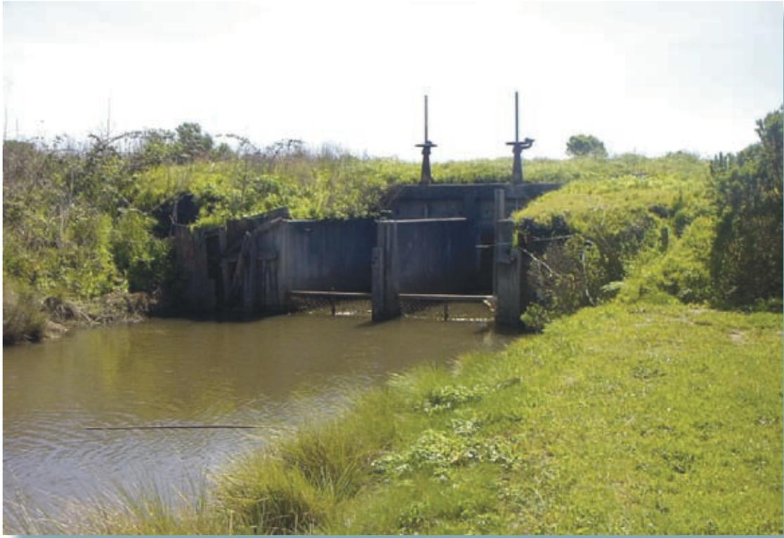
**Figure 24.** Tide gate separating Eureka Slough, Humboldt Bay, Humboldt County, California, and the drainage ditch that parallels California State Highway 101. The drainage ditch is in the foreground.
