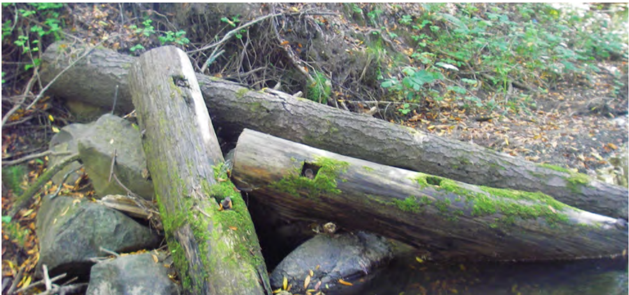
Artificial large wood structure bolted into boulders (Napa County).
