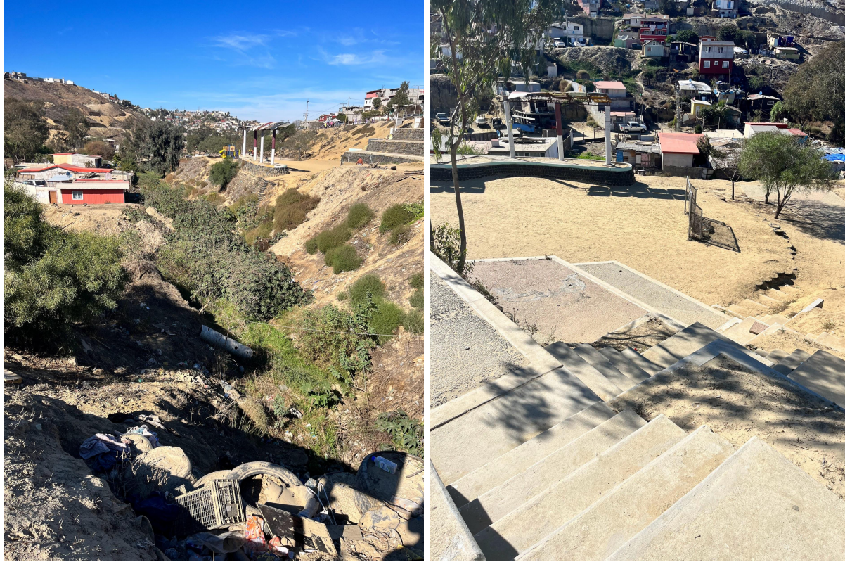
Figure 1-18 Taken from the road that cuts across the stream looking north into the riparian corridor of the stream. Noting the tires along the banks used to stabilize the bank from erosion. Figure 1-19 is taken from the street looking into the terraces of the Fronterizo park (32.491122, -117.082843.)
