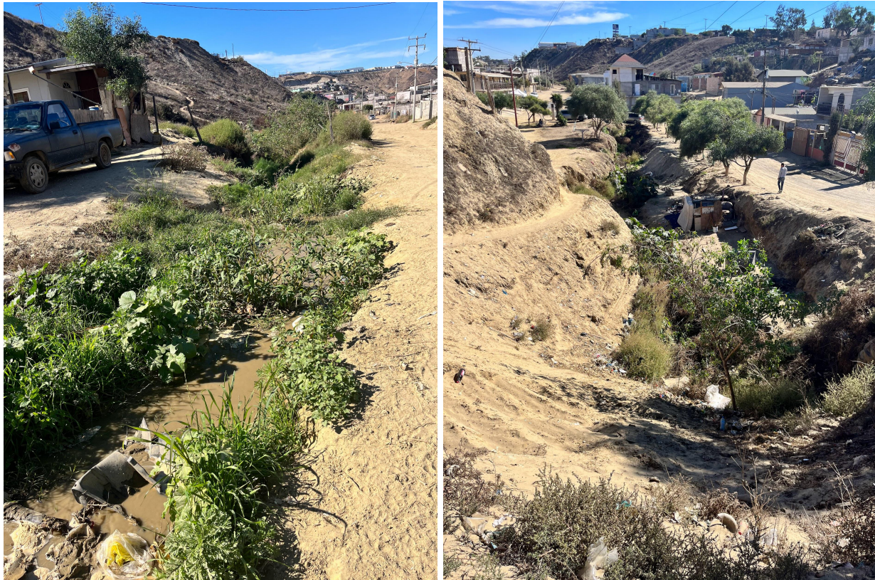
Figure 1-20 shows the streetscape of the region (32.487092,-117.078721). Figure 1-21 is taken from Calle Amanecer looking South into the stream. At this point the channel is not urbanized, Acacias were planted to line the banks of the stream.
