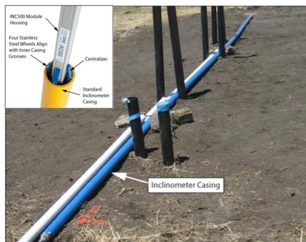
**Fig. 3. Inclinometer casing on ground surface prior to levee construction, and INC500 instrumentation detail.**
