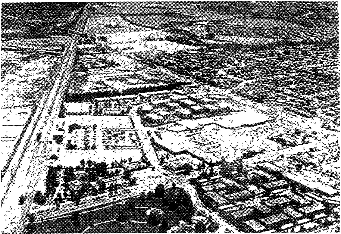
Photo 11.1. Union City Station Area
