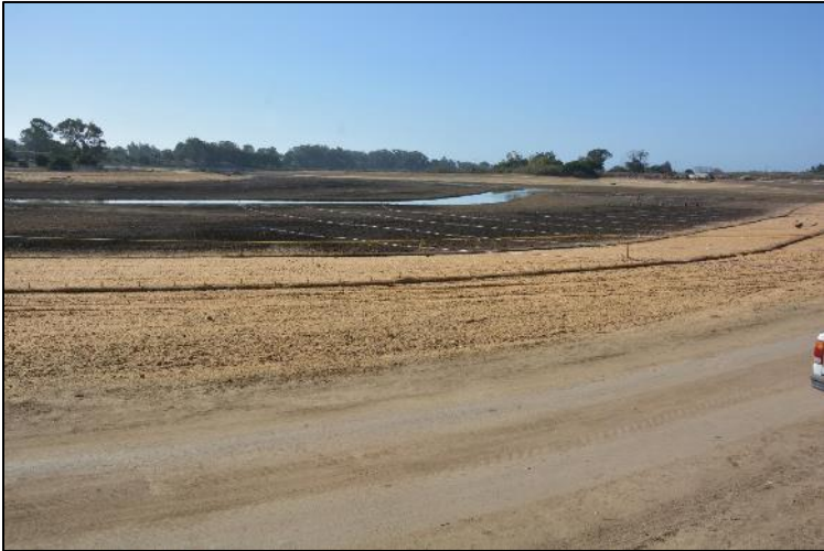
Baseline (post-grading) - October 2017
