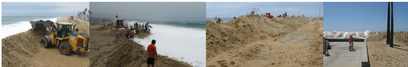
Figure 1. Anthropogenic berms such as these are constructed in the days and hours before an anticipated flood event in Southern California; they have been termed “event-type berms” by Gallien et al. (2014). (Color for this figure is available in the online version of this paper.)
