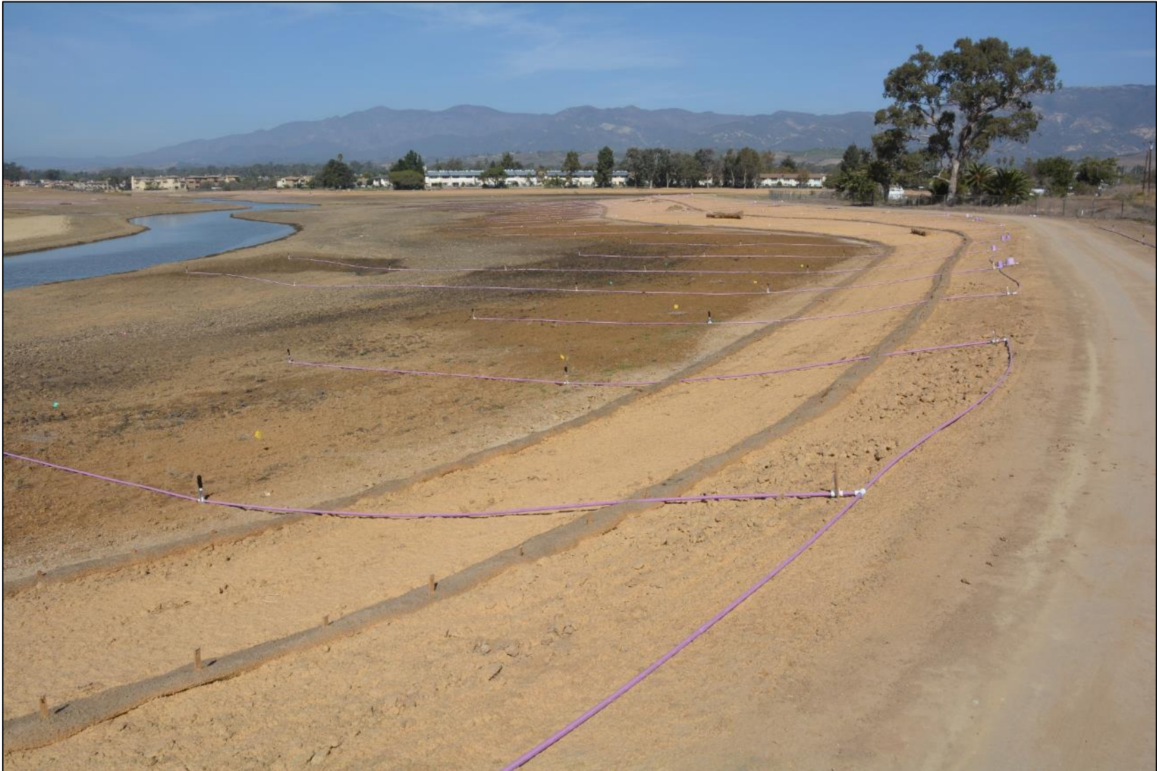
Baseline (post-grading) - October 2017
