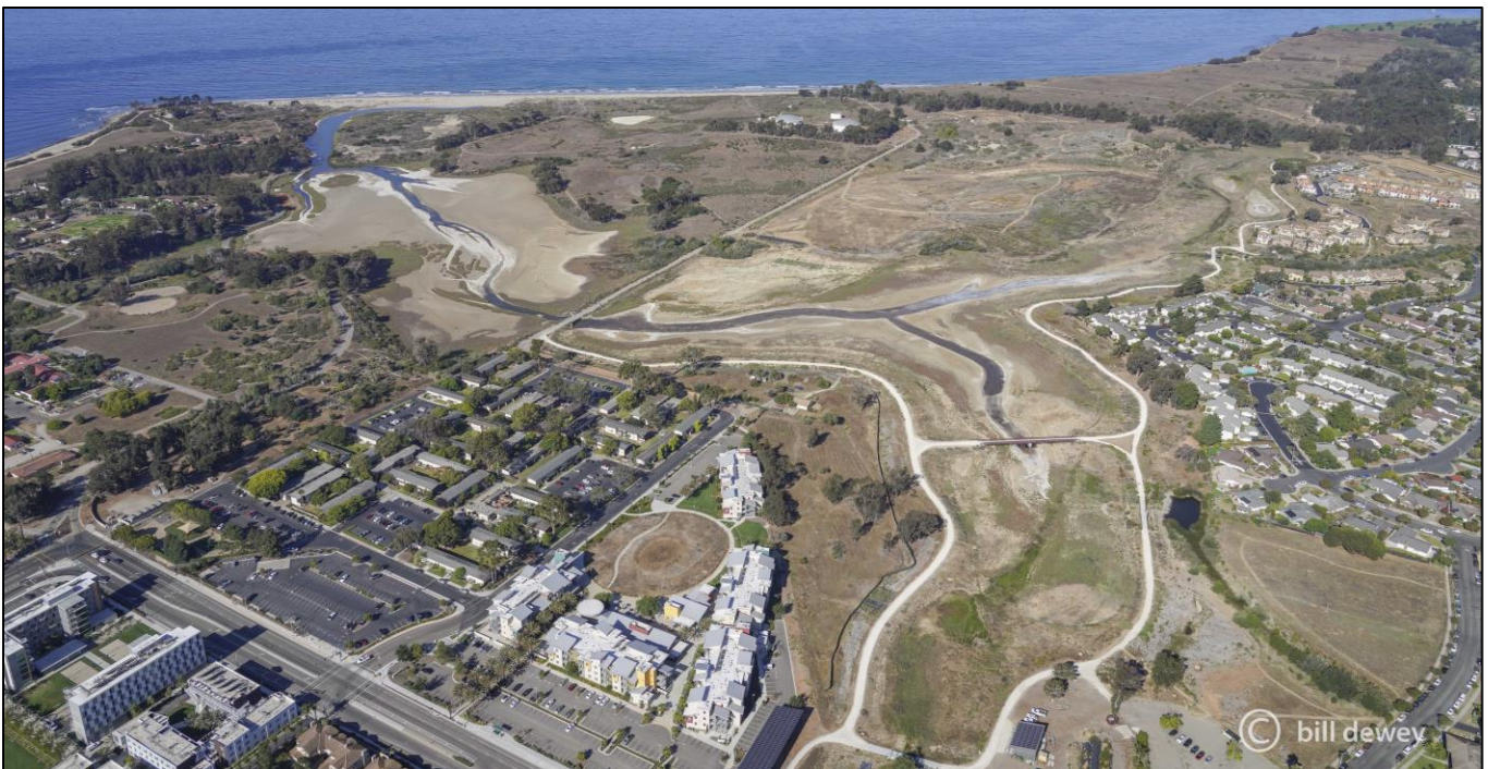
Figure 25. Aerial photos of North Campus Open Space by Bill Dewey. Top: December 2019 showing the high-water level; Bottom: August 2021 showing the low water level.
