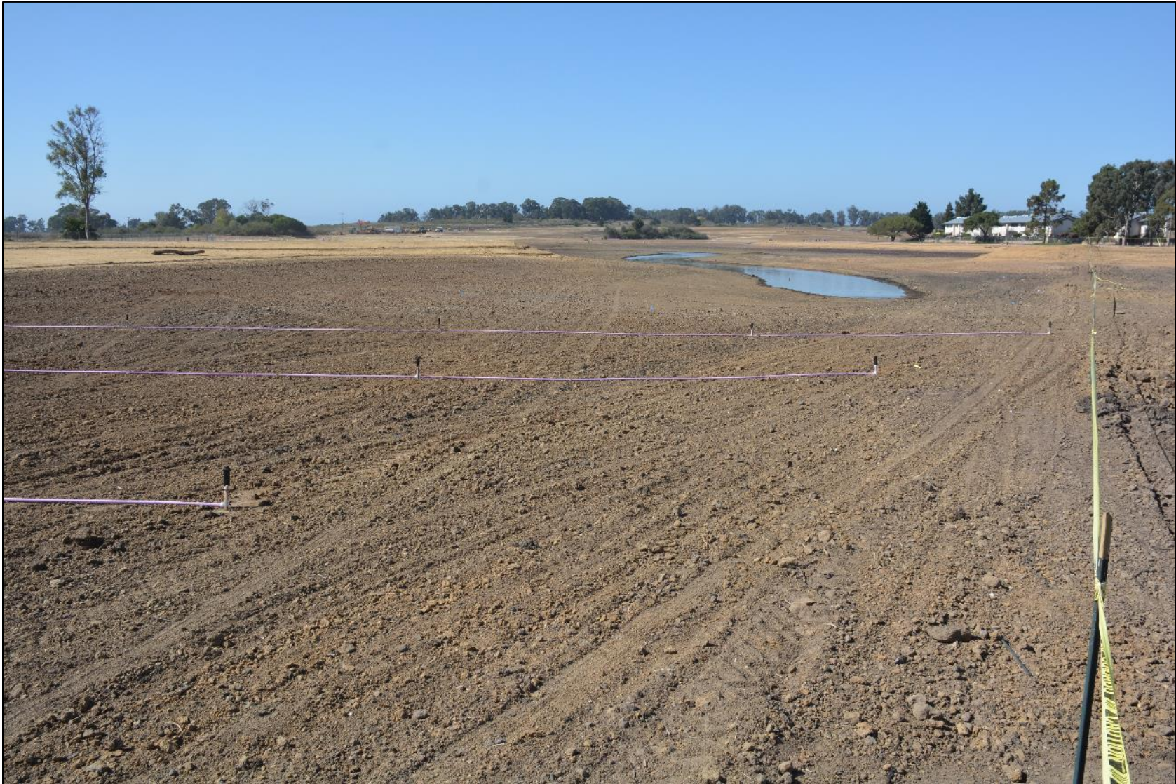
Baseline (post-grading) - October 2017
