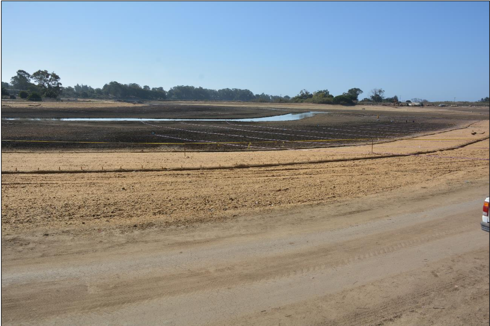
Baseline (post-grading) - October 2017
