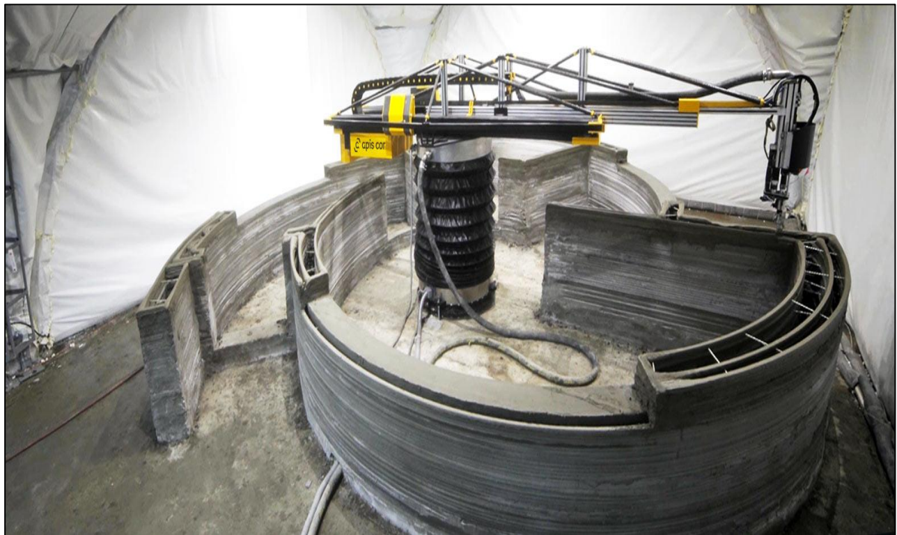
Figure 3.6: Apis Cor Crane Printer. [40]
