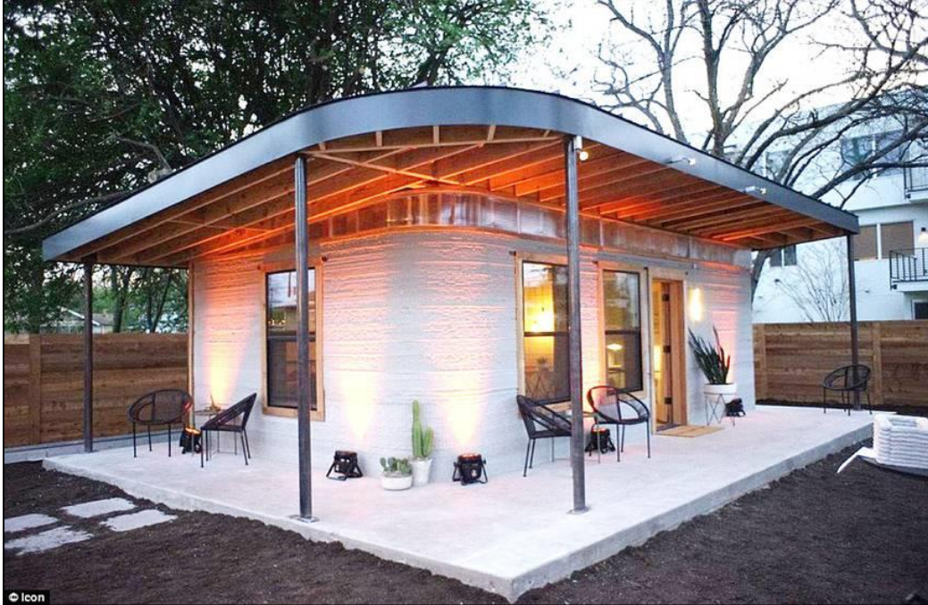
Figure 3.2: ICON® 3D Printed House [18]
