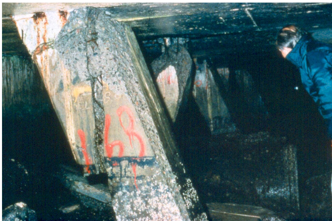
Figure 1-3: Damage to the battered piles that extended through the rock fill and liquefiable layers at the Port of Oakland after the 1989 Loma Prieta Earthquake. (Courtesy of John Egan, Geomatrix).
