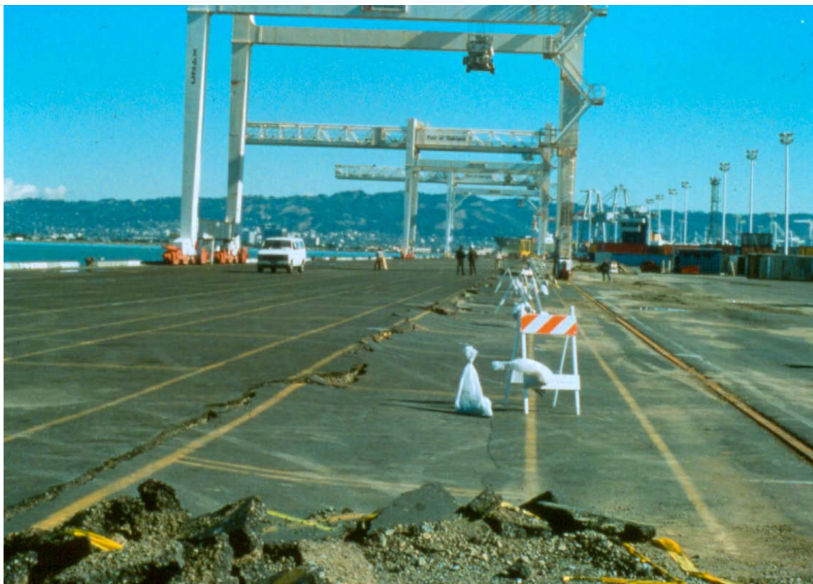
Figure 1-1: Top of the wharf structure at the Port of Oakland following the 1989 Loma Prieta earthquake. The cranes could not operate due to separation of the rails caused by extension of the wharf. (Courtesy of John Egan, Geomatrix).
