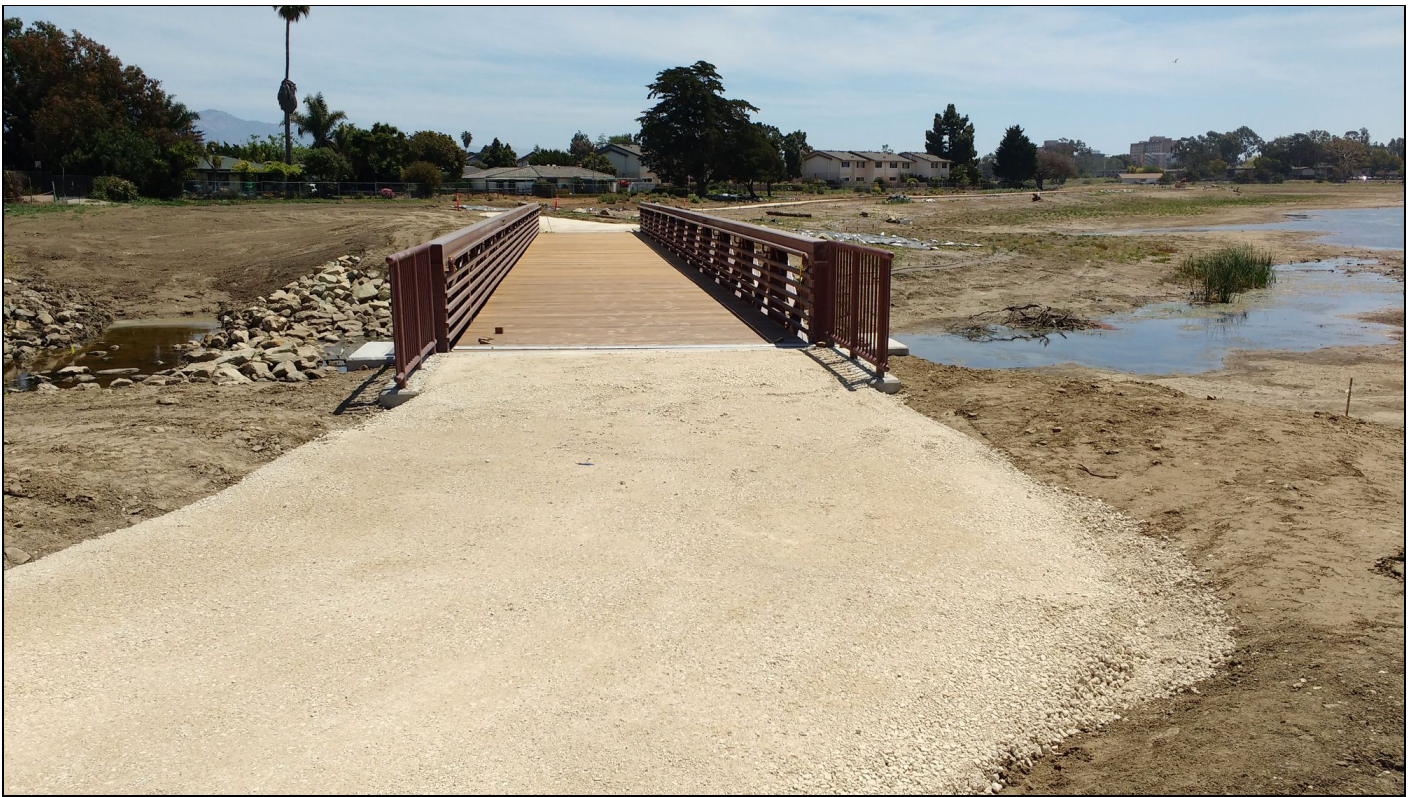
The trail and bridge over the Phelps Creek tributary of NCOS.
