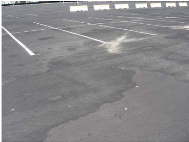
Figure 3: Photographs of Oil Stains and Evidence of Charcoal Use at Oakland Coliseum
