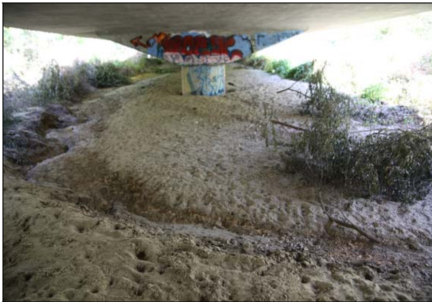
Figure 3a: Highway 68 underpass at El Toro Creek
