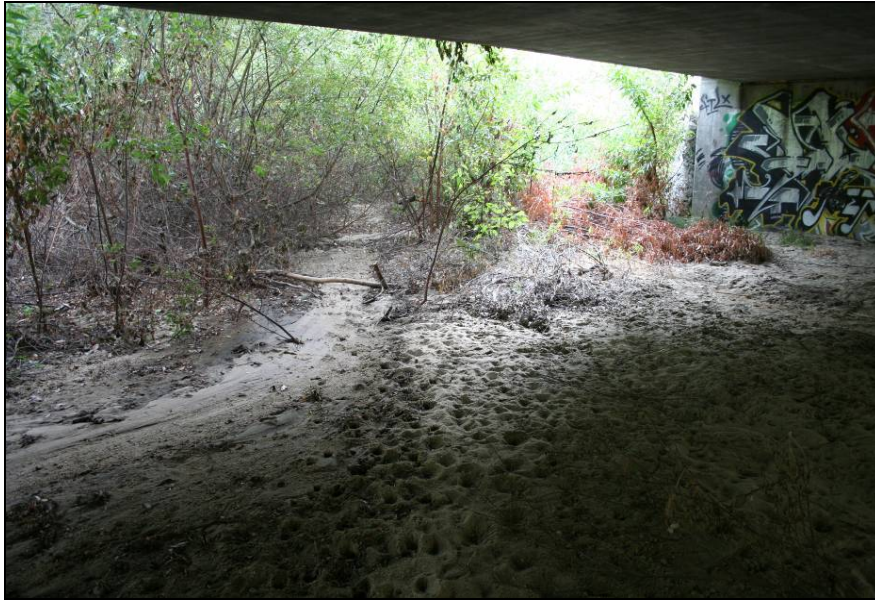
Figure 3b: Highway 68 underpass at El Toro Creek: east side
