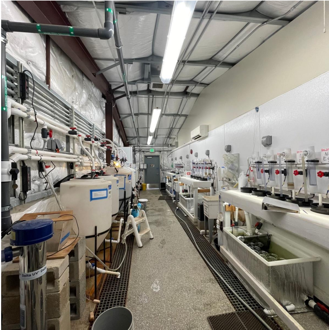
Figure 2.5 Egg and Live Prey Production Room at the FCCL. The room houses three independent incubation systems as shown in Figure 2.2. They can operate independently, and their water temperatures can be adjusted to meet the specific needs of different species such as Delta Smelt and Longfin Smelt.
