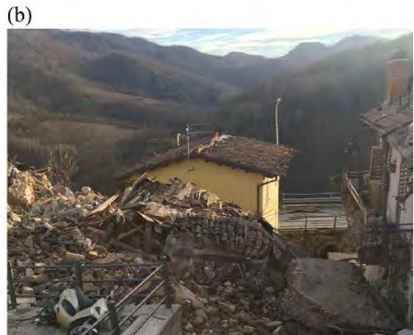
Figure 10. Masonry residential building: (a) after the first earthquake; and (b) after the sequence.
