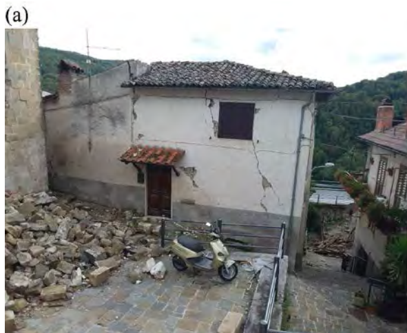
Figure 10. Masonry residential building: (a) after the first earthquake; and (b) after the sequence.
