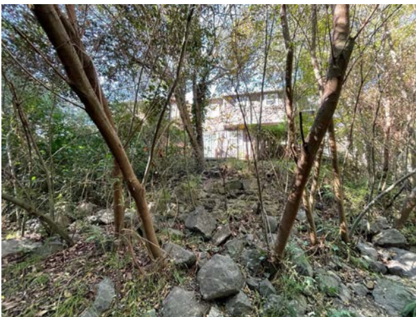
Photo 15. T3 facing right bank (SW)
