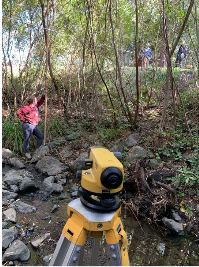
Photo 9. Right bank looking upstream (left bank in Figures 1, 2, 4, 5, and 6) while surveying at T3. Instrument is at second TP position.
