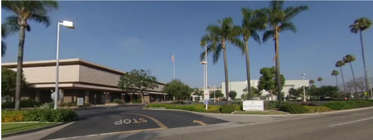
Figure 3.5. Entrance to MainPlace Mall looking towards JCPenney (Google Earth, 3/23/2021)
