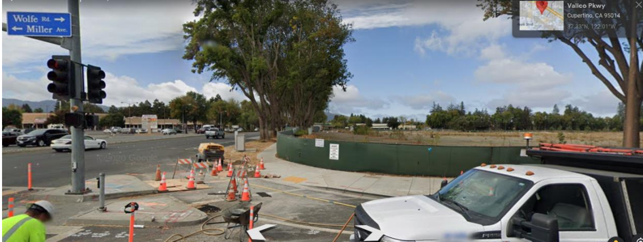
Figure 9.2. Wolfe Road and Miller Avenue, Vallco site under construction (Google Earth, 3/21/2021)
