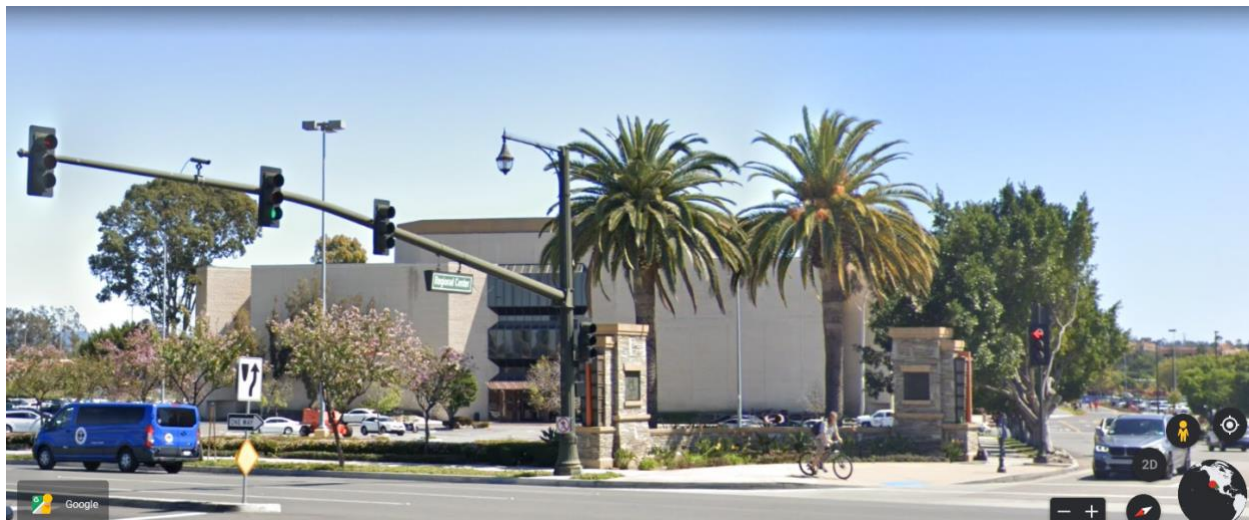
Figure 4.4. View of Laguna Hills Mall from El Toro Road (Google Earth, 3/4/2021)
