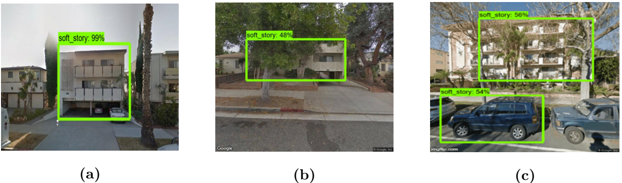
Figure 1.2. Soft-story detection with (a) non-blocked, (b) partially blocked, and (c) fully blocked images. (adapted from [40, 41])
