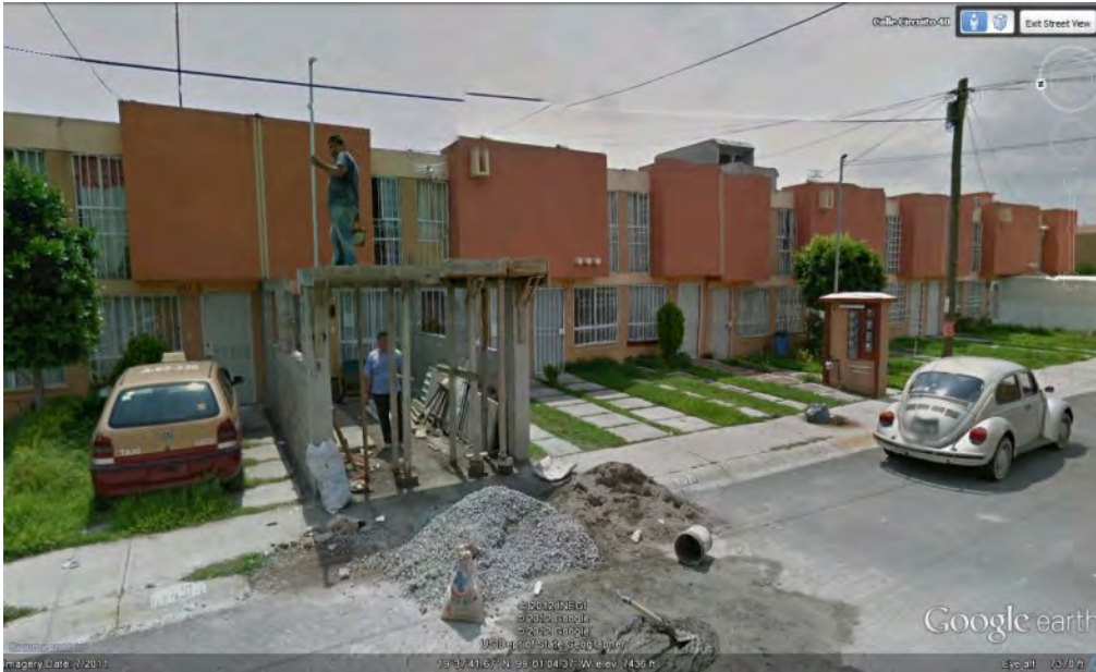
Figure 4.13 Reuse of parking space underway (Ecatepec, State of Mexico)
