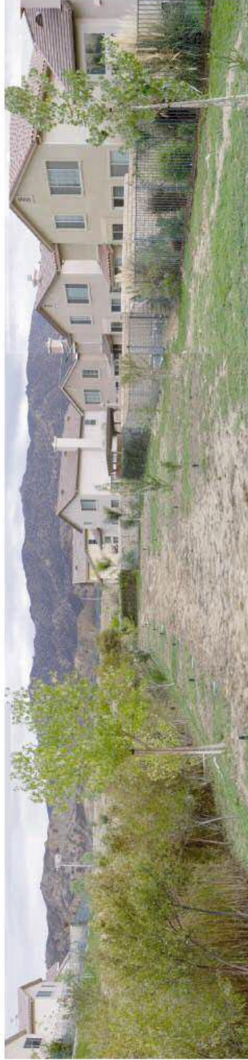
B Left Bank North View: The setback of the upper terrace illustrates the relationship between the constructed channel, the flood zone, residential back yards, and the protection of developing riparian habitat. The enclosure provides a protected common area, a view corridor and buffer zone that is not easily accessible. Pampas grass on adjacent private property (right) reveals the difficulties of limiting the introduction of exotic species in the future. Perhaps future planning guidelines for Homeowners Associations should address limiting invasive exotics near riparian corridors.
