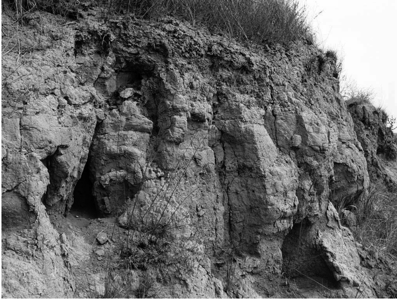
Figure 1.4. Dabuzishan Town Remains: Rammed-Earth Wall, Eastern Section
