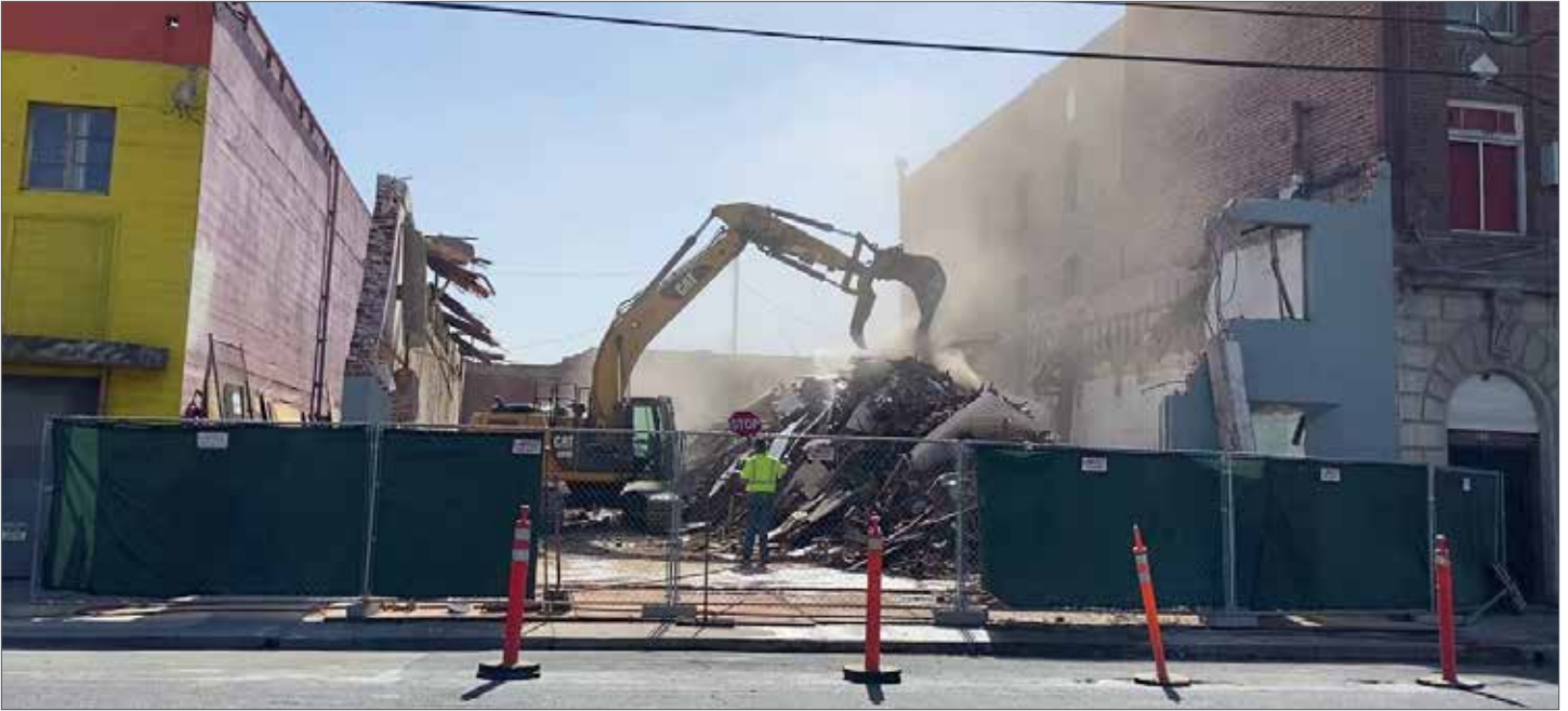
Demolition of Razil Social Cub, a culturally significant building in Stockton's historic Little Manila district, after financing could not be secured for structural repairs. Photo credit: Little Manila Rising
