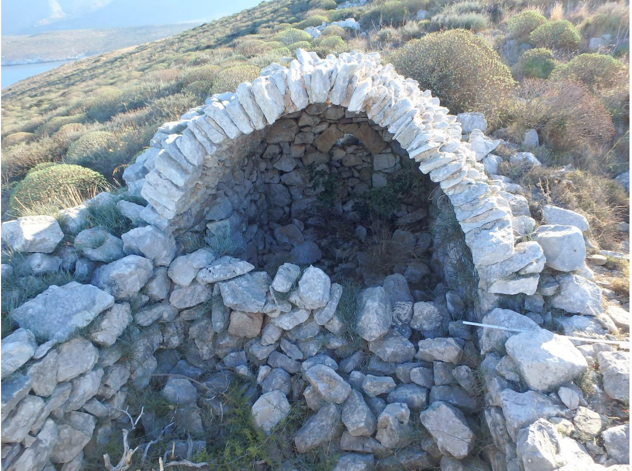
Figure 109: View of interior of church looking east near Tigani. (Photo: M. Pawlowski)
