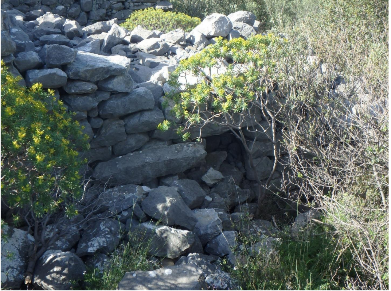
Figure 192: Lower doorway on western wall of lowest phase of House 8. (Photo: M. Pawlowski)
