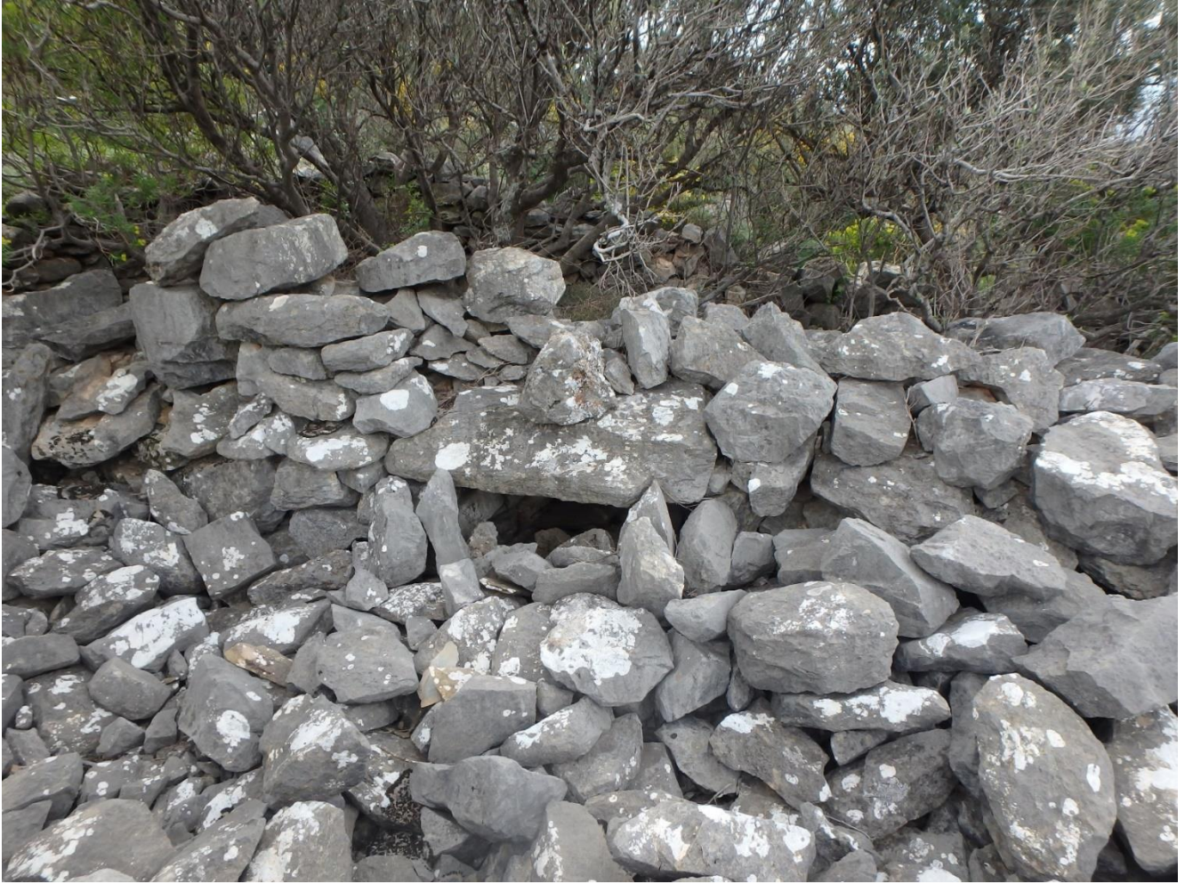
Figure 178: View of lower entrance from the north. (Photo: M. Pawlowski)
