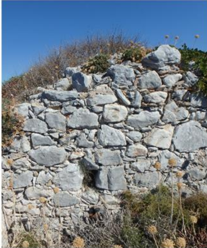
Figure 118: Detail of wall construction from Tigani. (Photo: M. Pawlowski)
