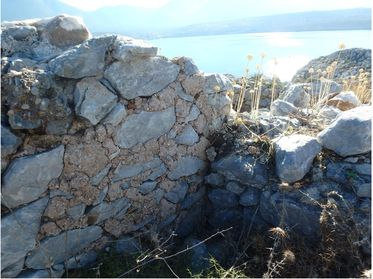
Figure 125: East wall of Tower B at Tigani. (Photo: M. Pawlowski)
