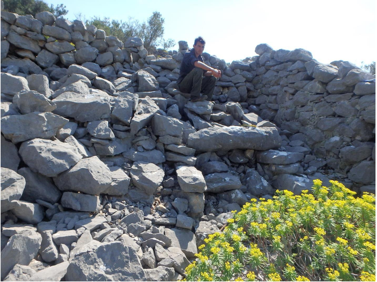
Figure 86: Large doorway to west of Marathos. (Photo: M. Pawlowski)
