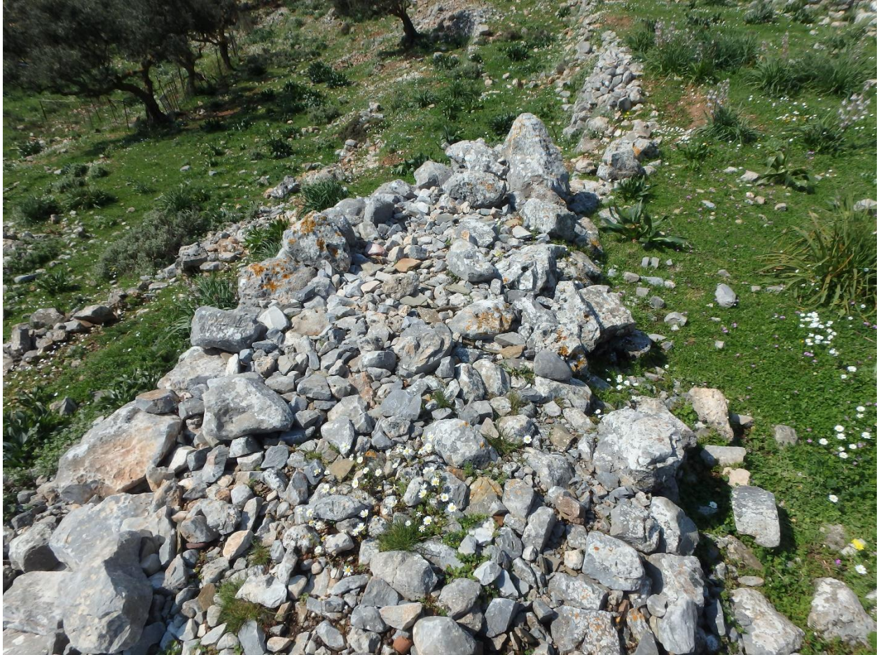
Figure 41: View of bulwark from above. (Photo: M. Pawlowski)
