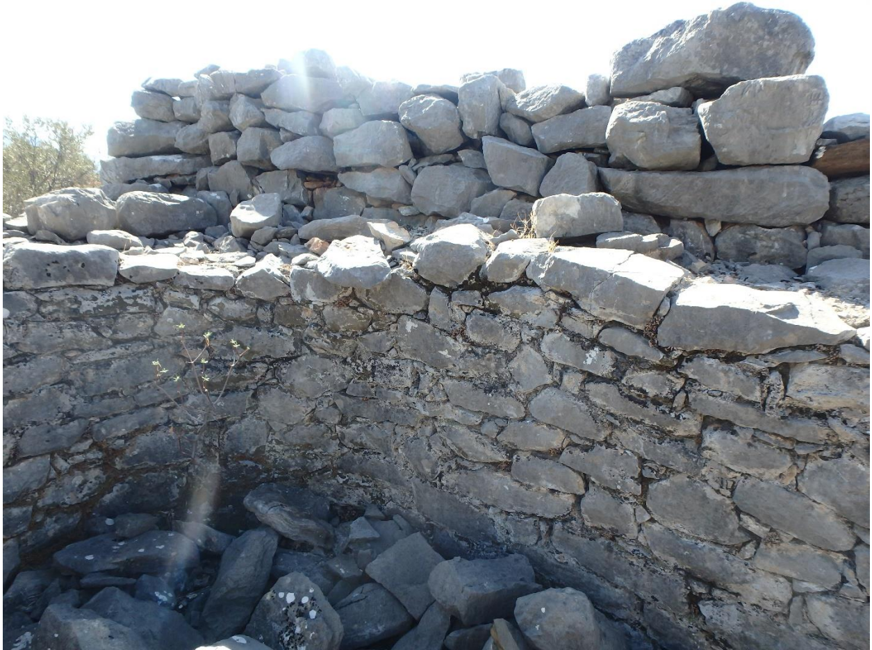
Figure 92: Detail of interior well of cistern. (Photo: M. Pawlowski)
