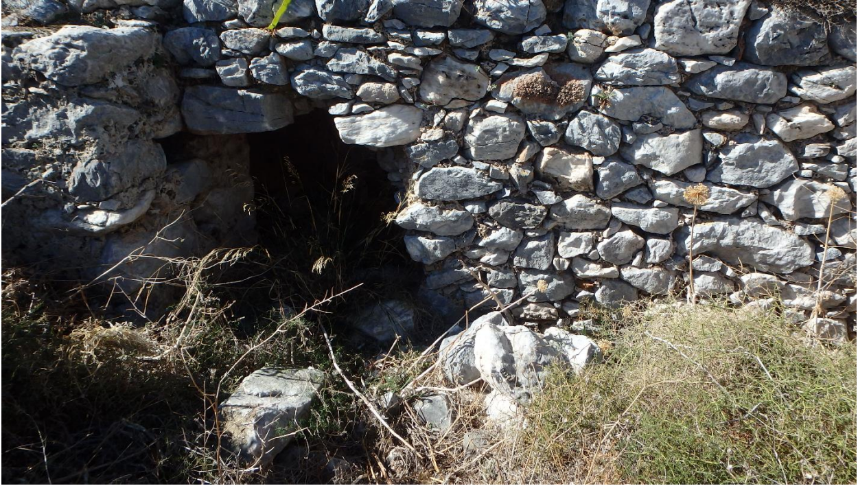
Figure 112: Interior “doorway” to cistern in House 4 at Tigani. (Photo: M. Pawlowski)
