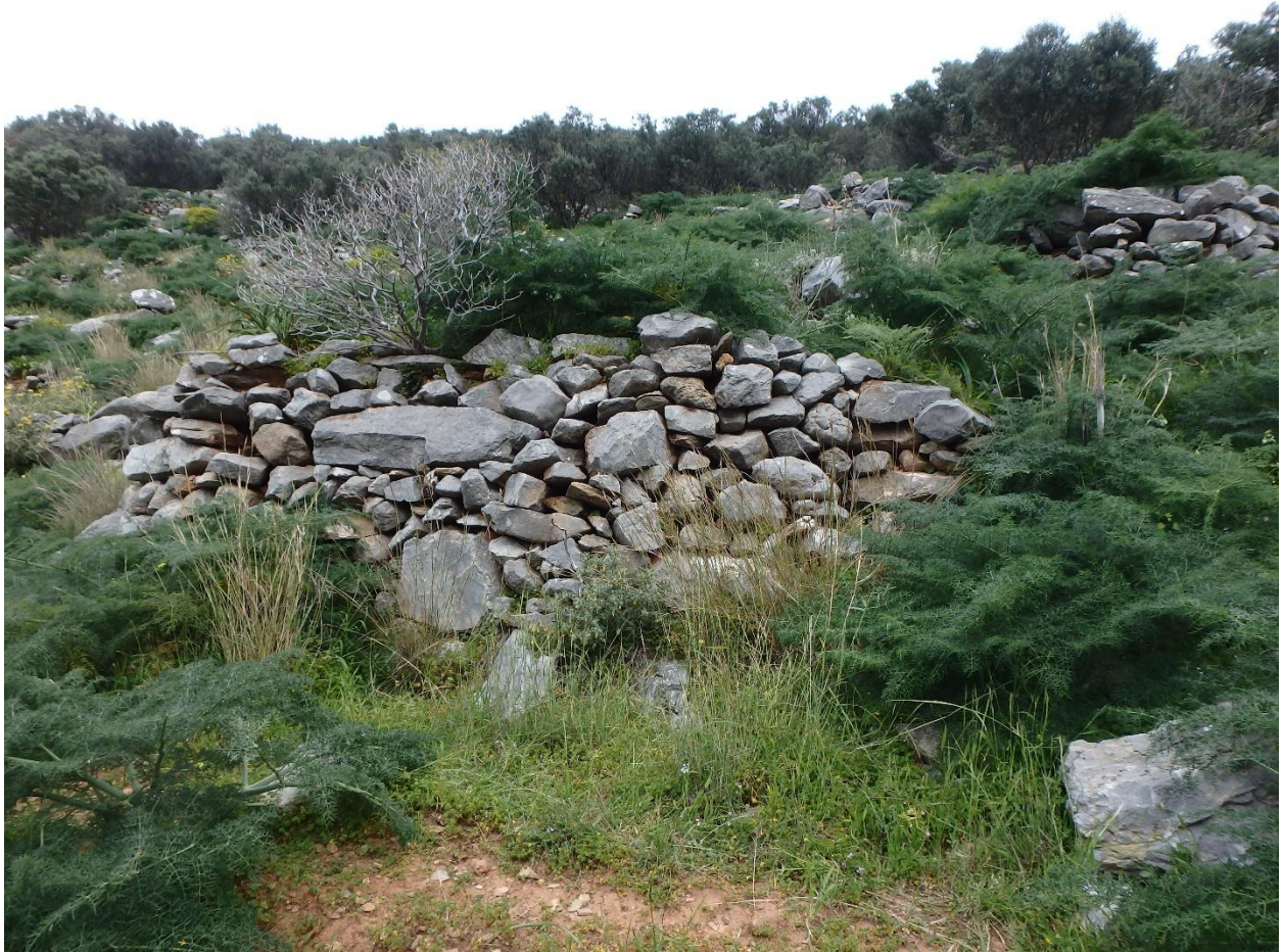
Figure 77: Example of construction from past Zone C, Marathos. (Photo: M. Pawlowski)
