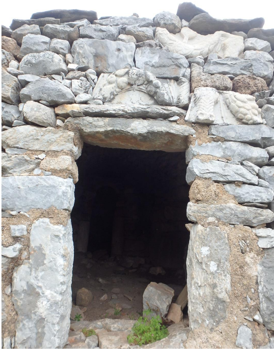
Figure 49: Pieces of marble spolia above western doorway on Hagios Philippos, Marathos. (Photo: M. Pawlowski)
