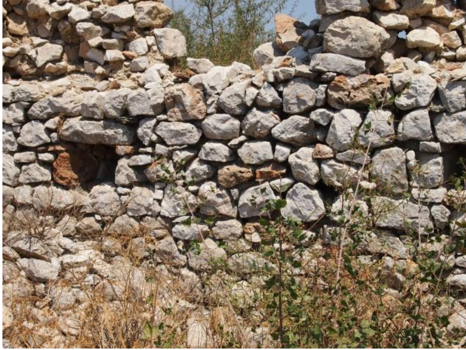
Figure 117: Detail of wall from Karyoupolis. (Photo: P. Katsafados)
