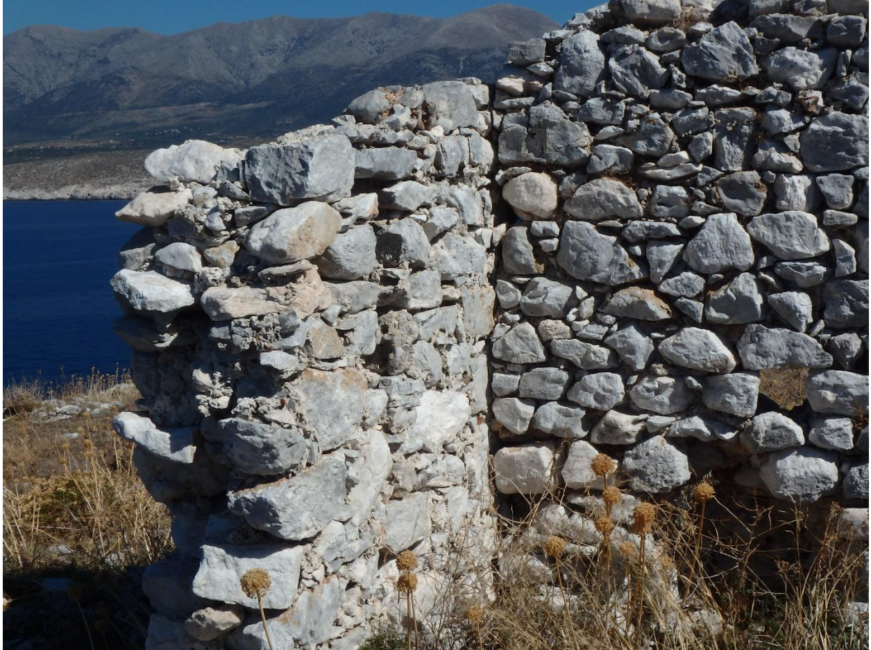
Figure 115: View of walls of House 5 at Tigani from southwest. (Photo: M. Pawlowski)
