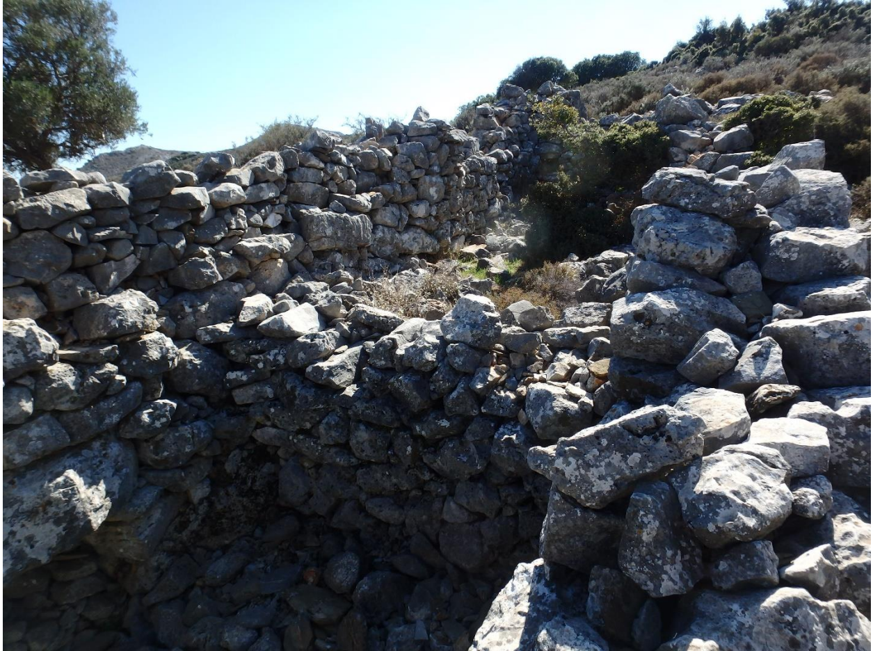
Figure 29: View of House 5, Sarania from the west. (Photo: M. Pawlowski)
