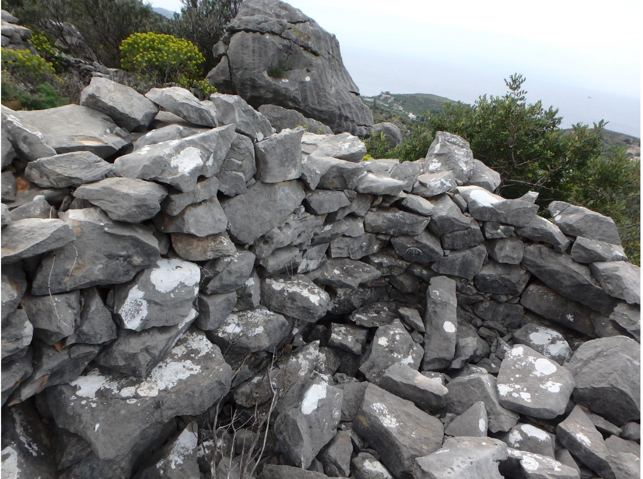
Figure 65: View of joist hangars from inside House 2, Marathos. (Photo: M. Pawlowski)
