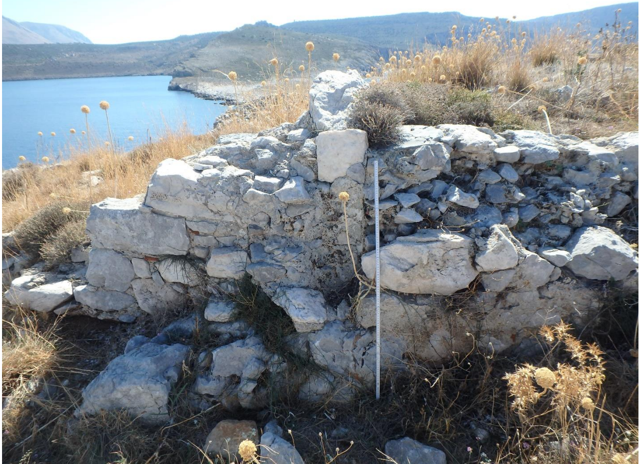
Figure 123: View of interior of south wall of gate at Tigani. (Photo: M. Pawlowski)
