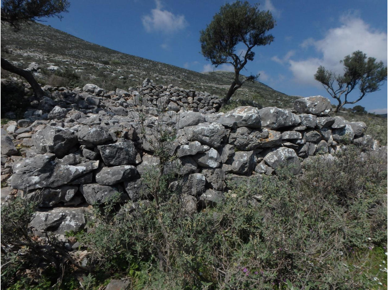
Figure 175: View of House 17 from the east. (Photo: M. Pawlowski)
