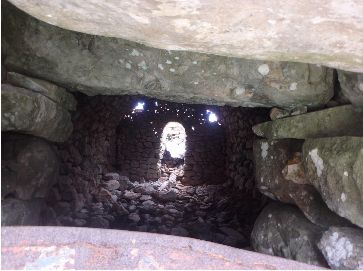
Figure 22: View of masonry icon screen in Hagios Georgios, Sarania. (Photo: M. Pawlowski)
