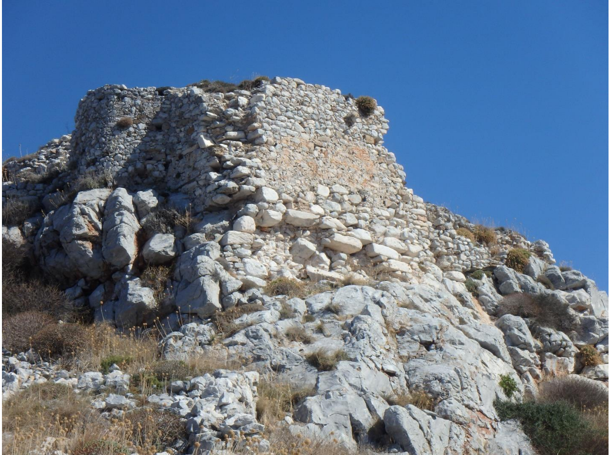
Figure 124: View of Tower C at Tigani from southwest. (Photo: M. Pawlowski)
