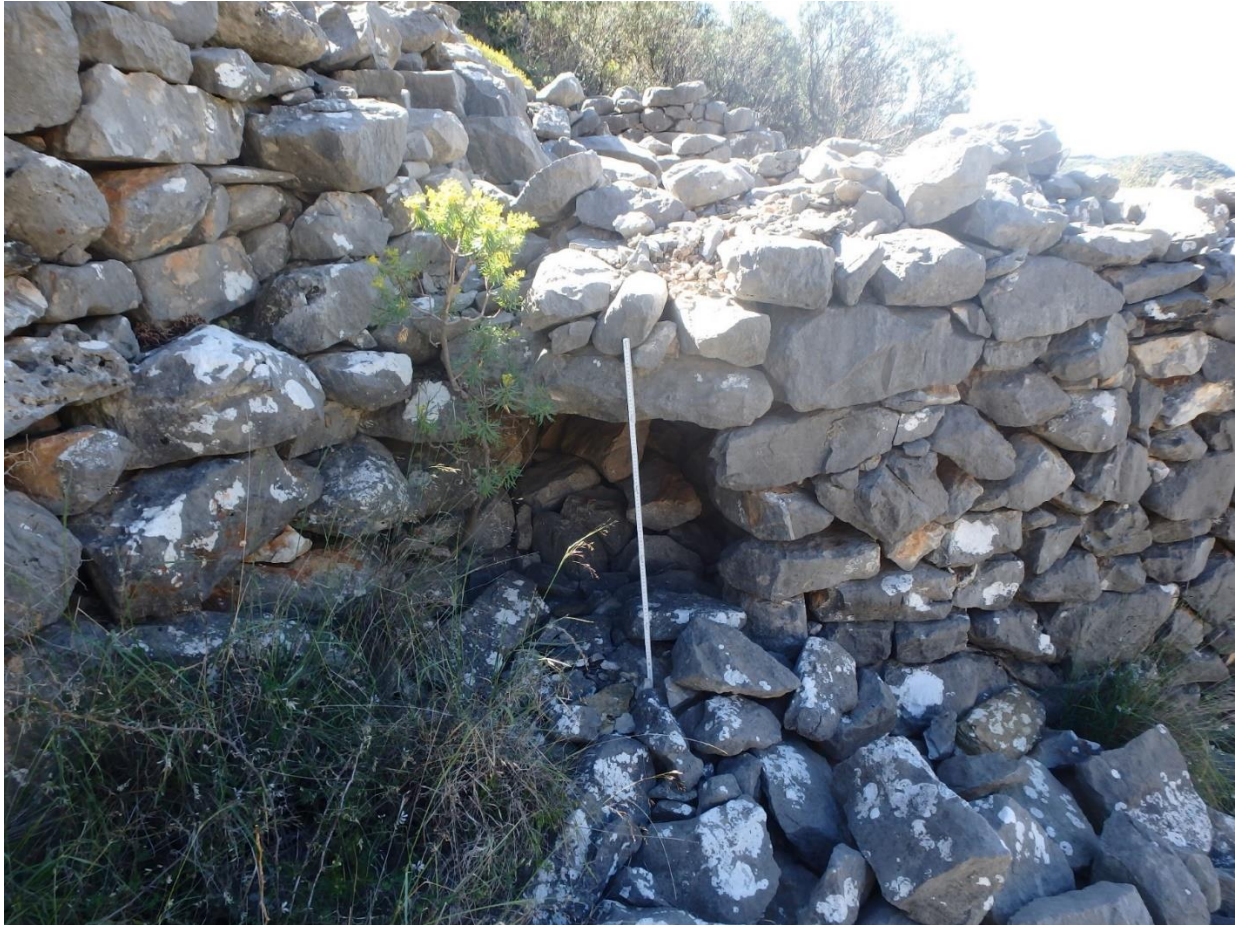
Figure 206: North doorway of House 15. (Photo: M. Pawlowski)
