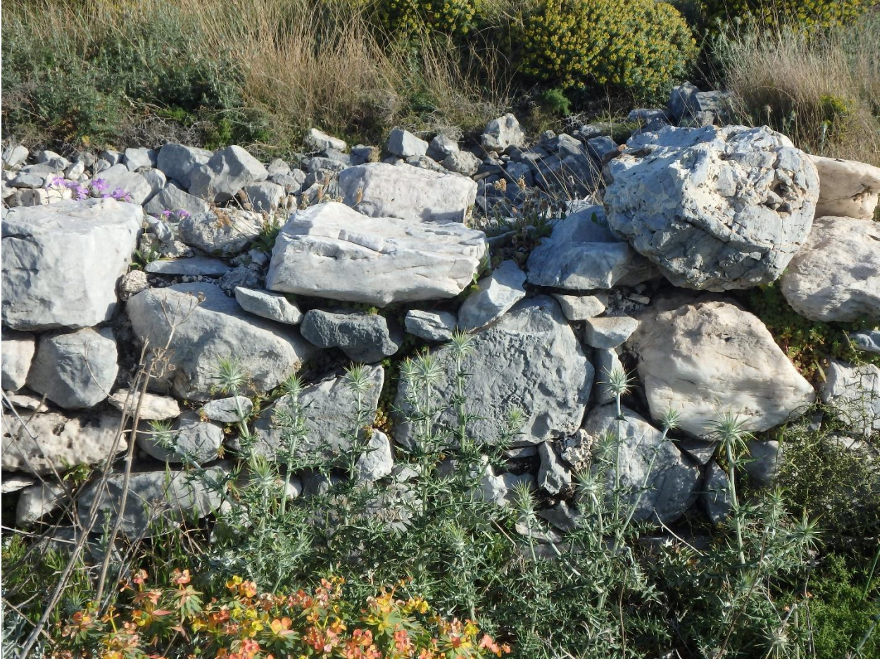
Figure 238: Detail of masonry from House 2. (Photo: M. Pawlowski)
