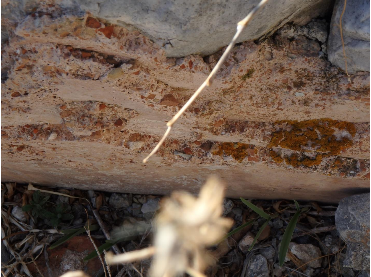
Figure 122: Final plaster layers in cistern at Tigani. (Photo: M. Pawlowski)
