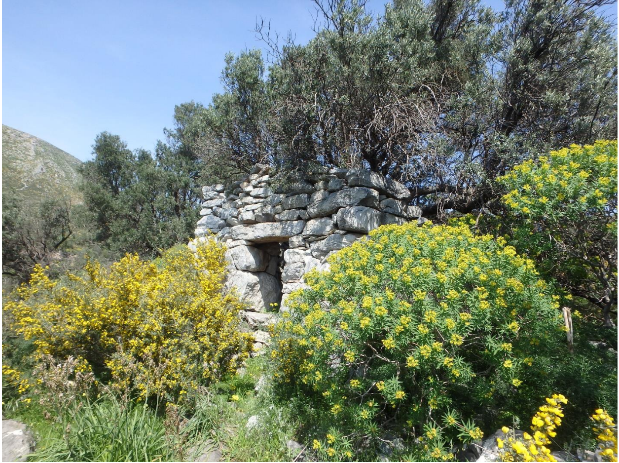
Figure 62: View of Church C, Marathos from southwest. (Photo: M. Pawlowski)
