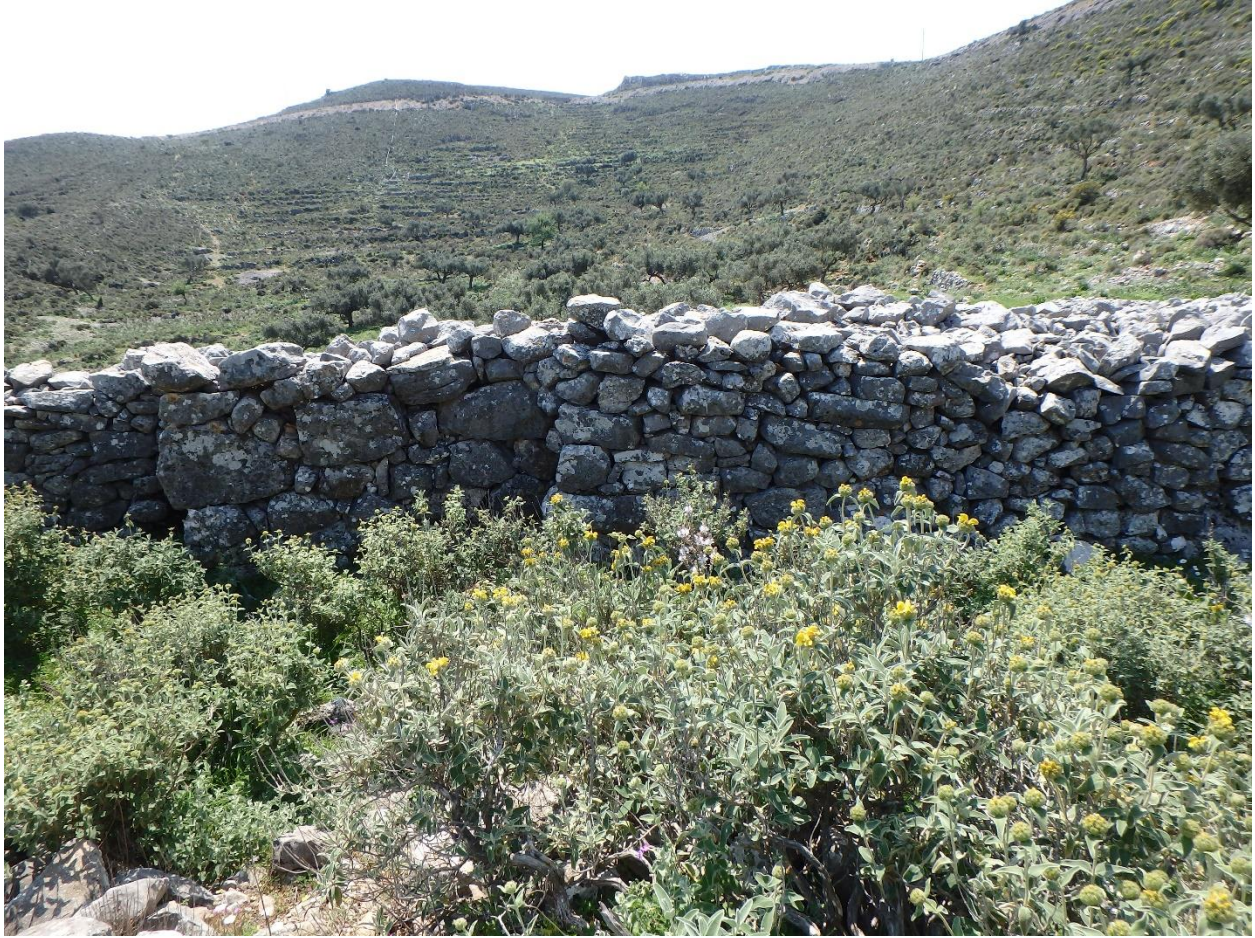
Figure 172: House 15 from the north. (Photo: M. Pawlowski)
