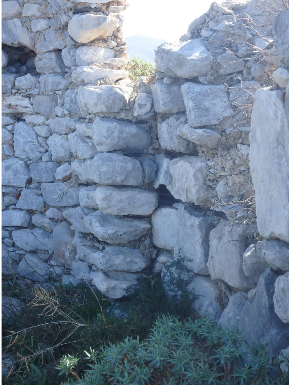
Figure 105: View of apse and south wall from the west. (Photo: M. Pawlowski)
