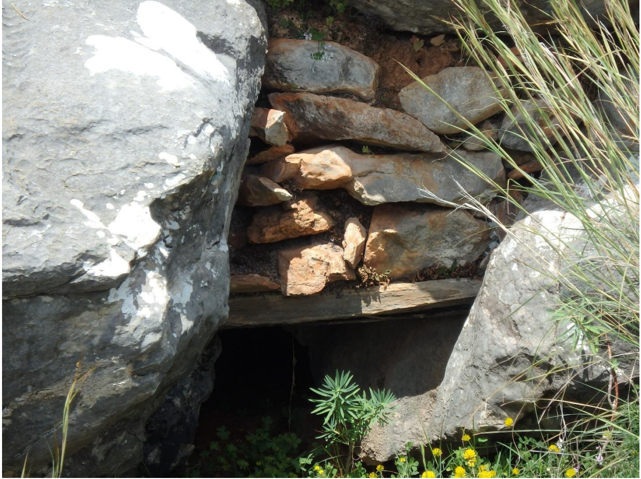
Figure 82: Drain north of Cistern H. (Photo: M. Pawlowski)
