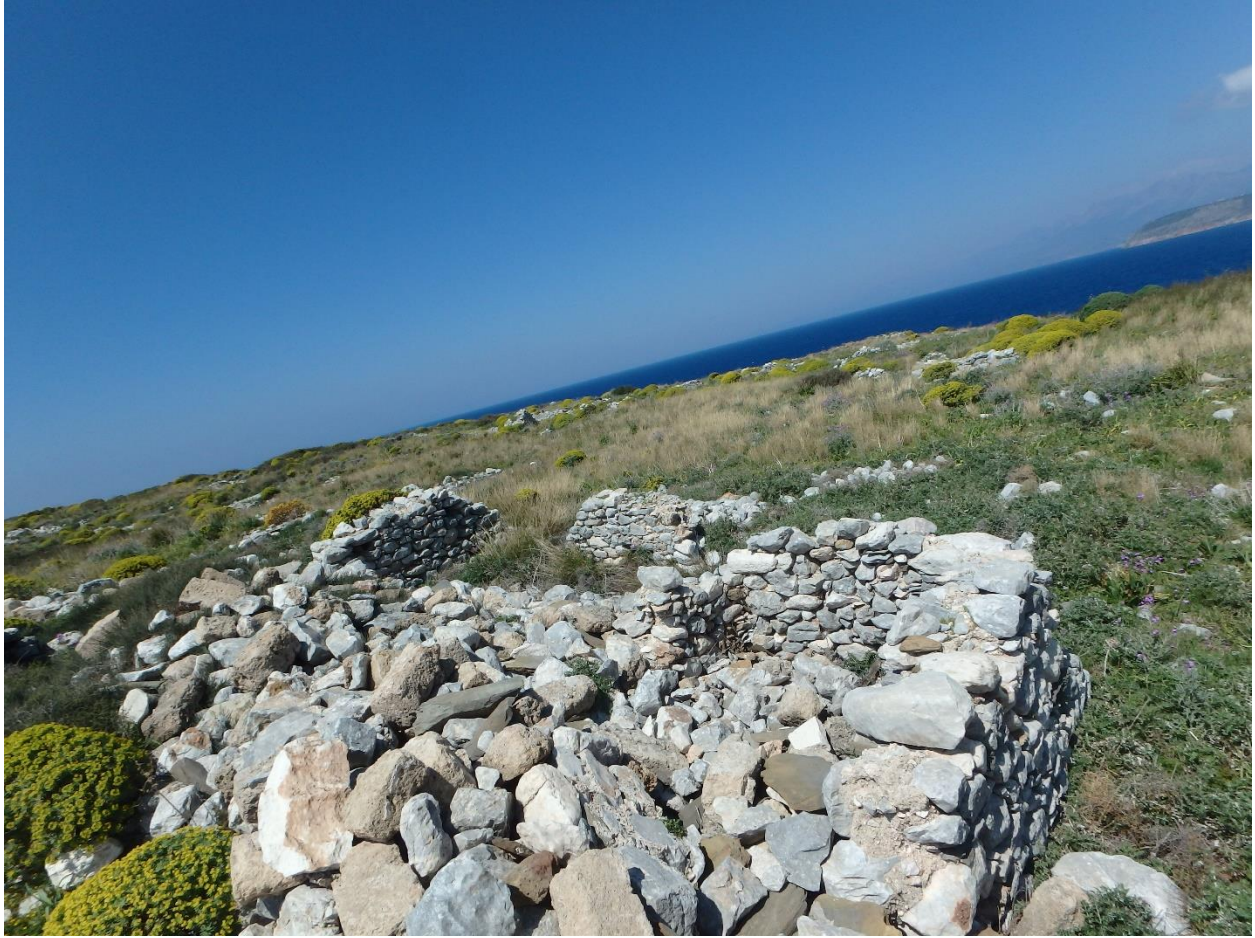
Figure 247: View of House 7 from the south. (Photo: M. Pawlowski)
