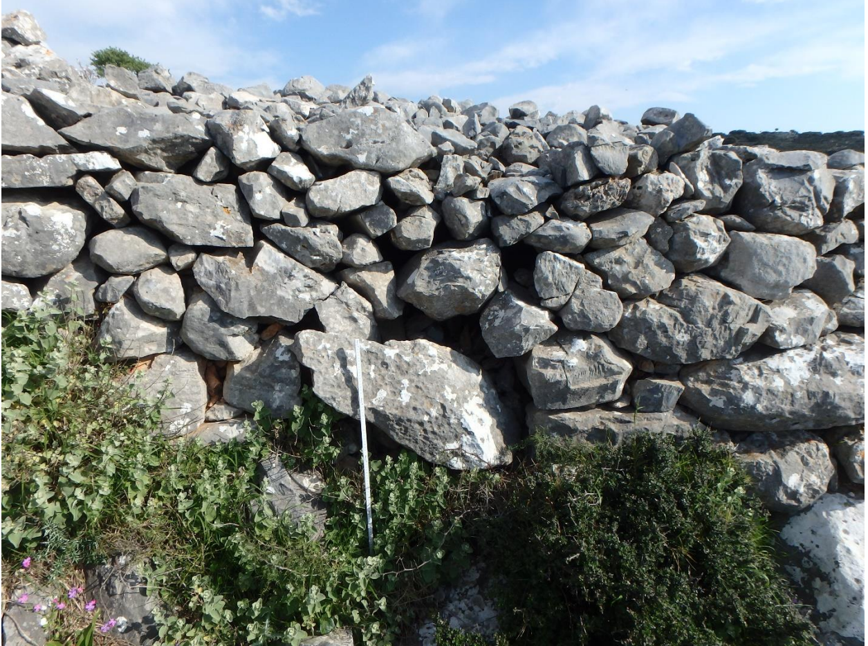
Figure 164: Collapsed doorway of House 11. (Photo: M. Pawlowski)
