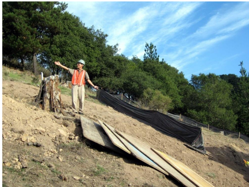
Figure 3-51. Trench TR0 after filled, and location of trench TR1
