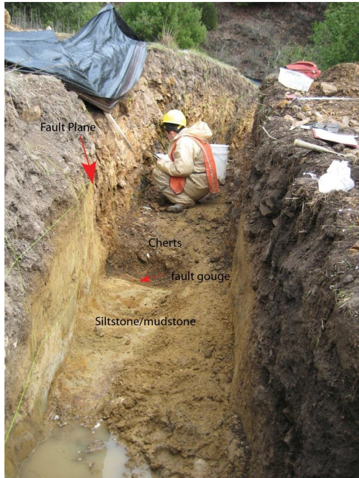
Figure 3-63. West view to NUMO TR3. Note the sharp fault contact between the Orinda and Claremont Formations
