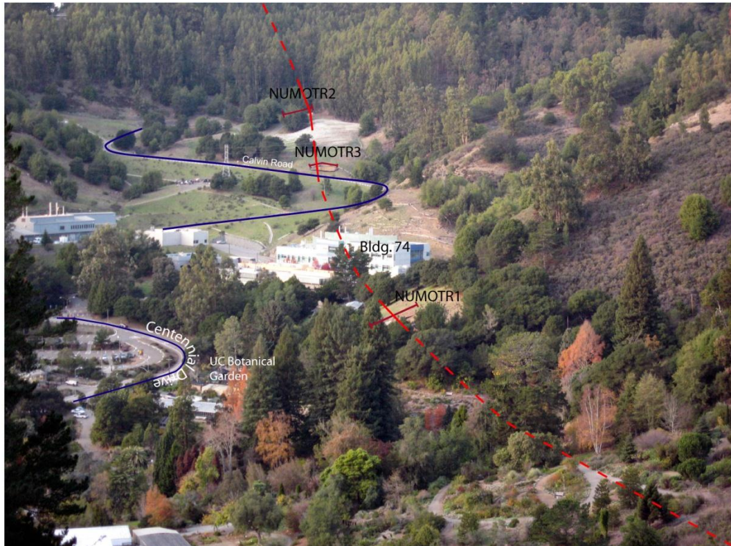
Figure 3-52. View from the Fire Trail of three open NUMO trenches. The lengths of NUMOTR01 and TR02 are approximate. Centennial Road and Building 74 are used as point of reference.
