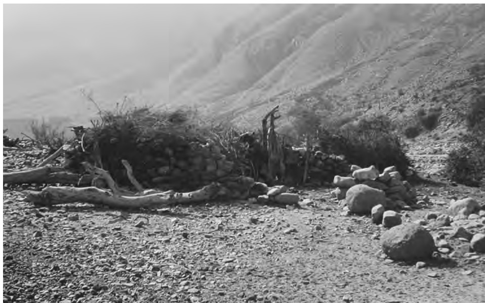
Figure 5. Modern residential structure located in the Tierras Blancas River Valley approximately one kilometer downstream (west) from Marcaya.
