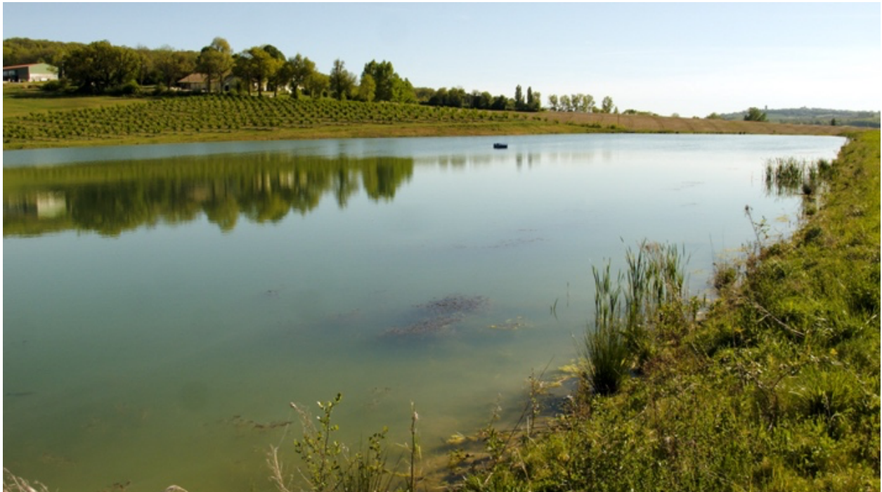
Figure 3.9. Second-generation, 50,000 m 3 retention pond in the Commune of Montflaquin, with recently planted hazelnut orchard in the background, each tree roughly the size of a soccer ball.
