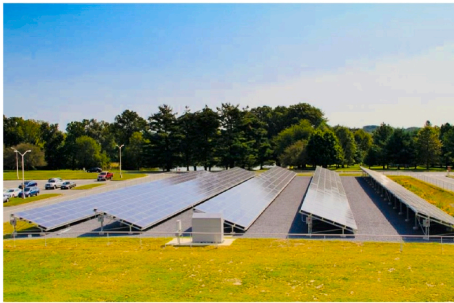
Fig. 7. NIST-ground array with 1152 PV modules for power modeling test.
