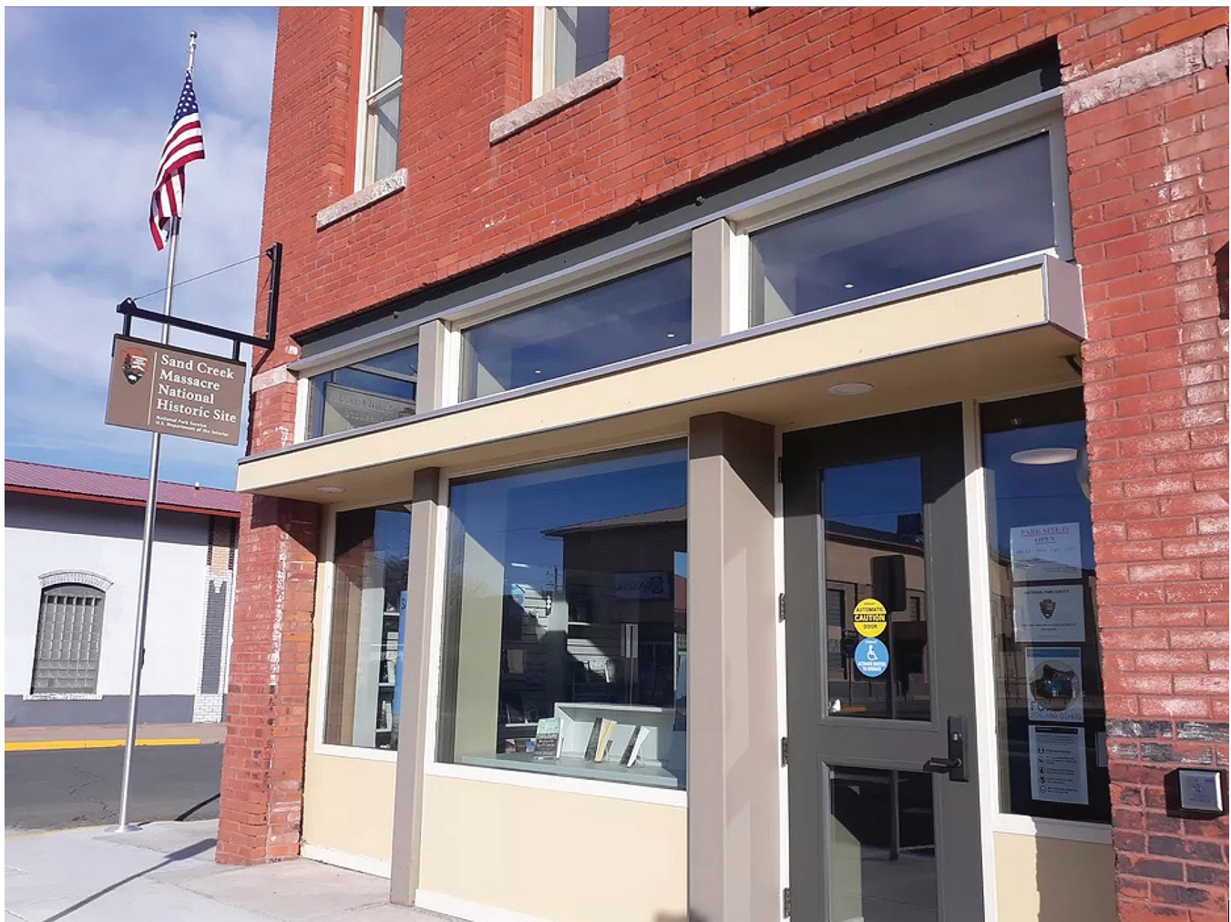
FIGURE 5. The Sand Creek Massacre Foundation in Eads, Colorado. ALEXA ROBERTS
