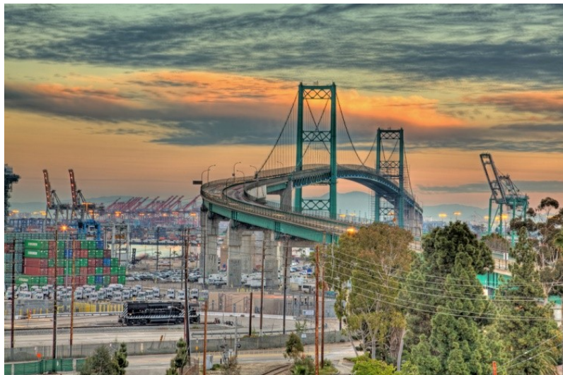
Figure 2.31: Vincent Thomas Bridge
